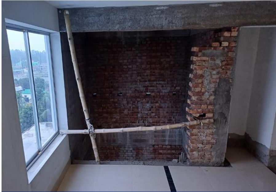
Falling hazard from lift core & 1 st floor
