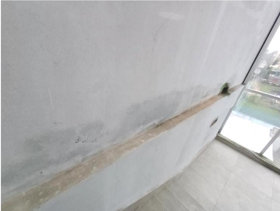
Dampness on brick wall
