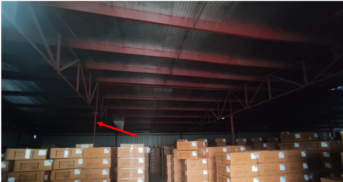
Slender pipe column (63mm steel pipe) at the center of truss
