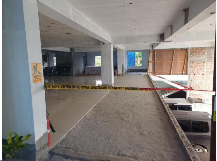
Falling hazard from lift core & 1 st floor
