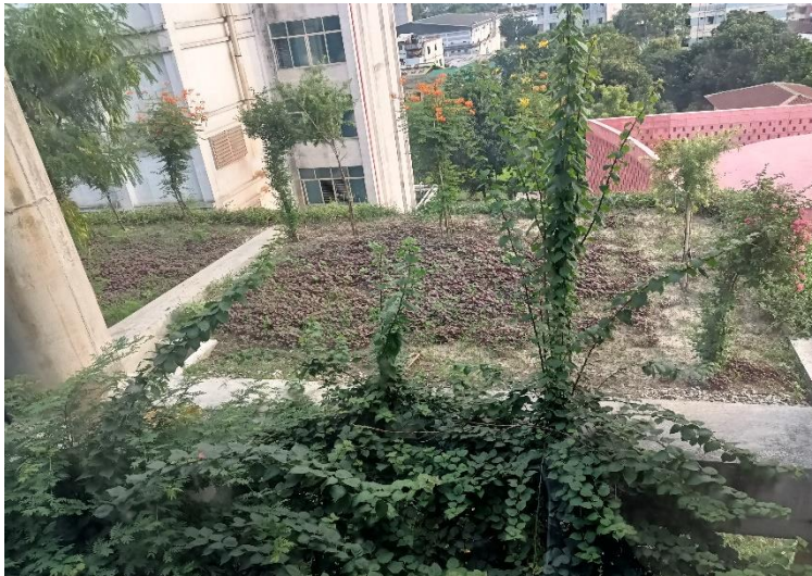
Garden at cantilever portion
