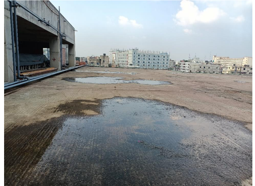
Sign of water clogging on the roof
