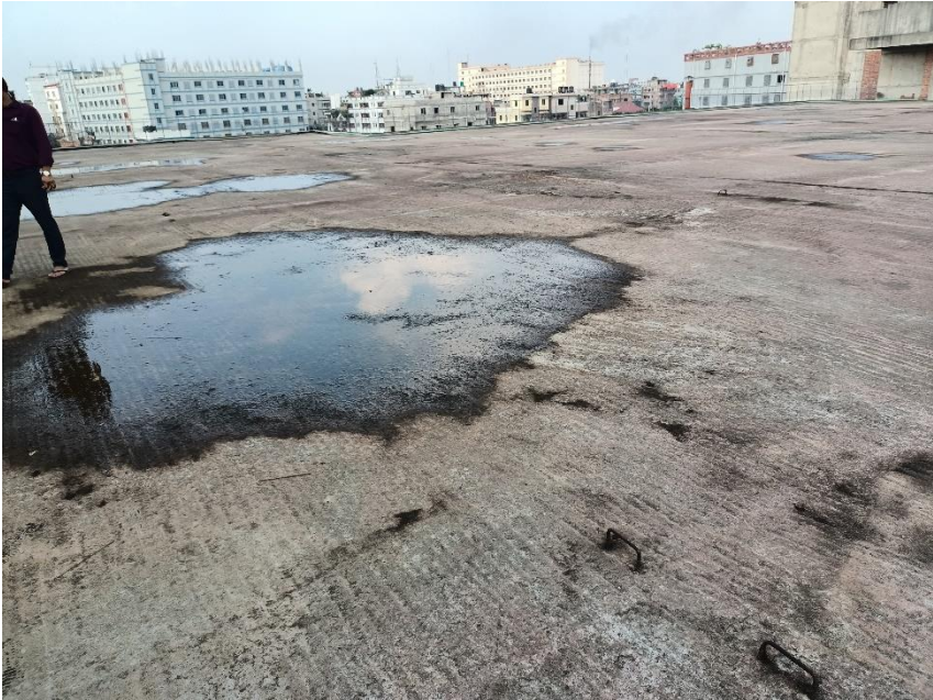
Sign of water clogging on the roof
