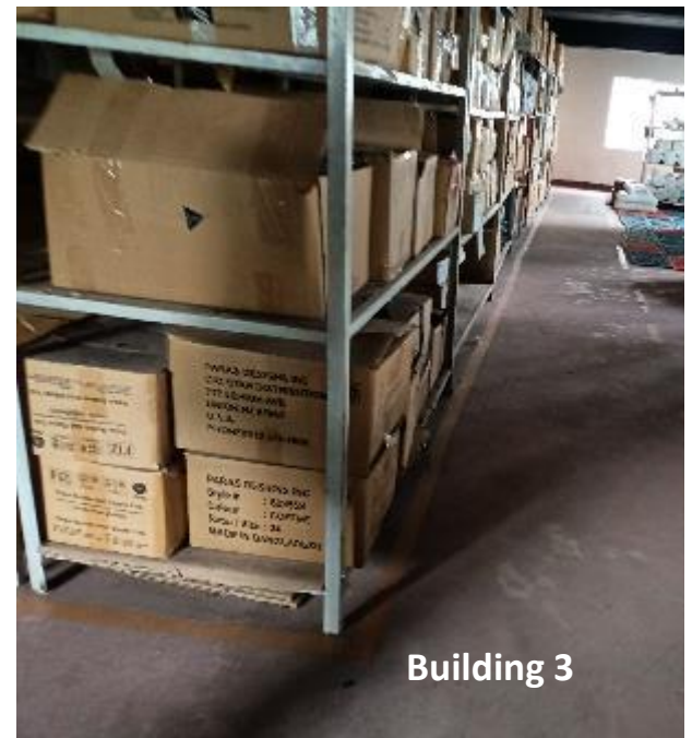
Plastic water tank & storage racks not anchored or braced
