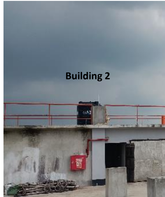
Plastic water tank & storage racks not anchored or braced
