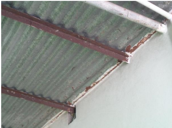
Steel angle member resting on the brick wall
