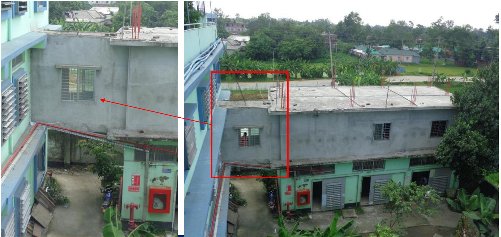
Main factory building and utility building structurally connected by slab
