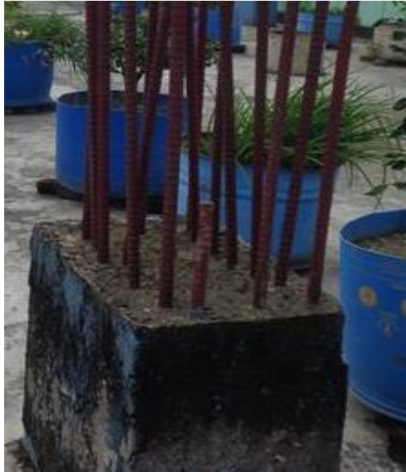
Exposed rebar on roof to confirm quantity
