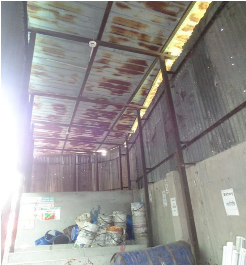
ETP dry sludge storeroom farming system.
