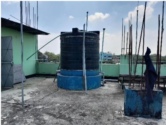
Undocumented water tank and telecom mast at roof
