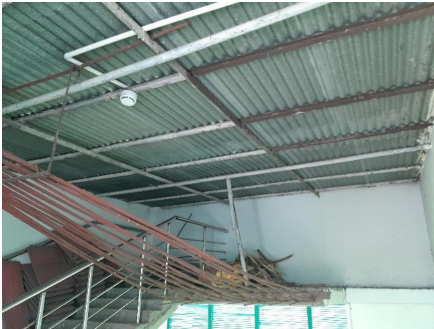
Non engineered staircase roof
