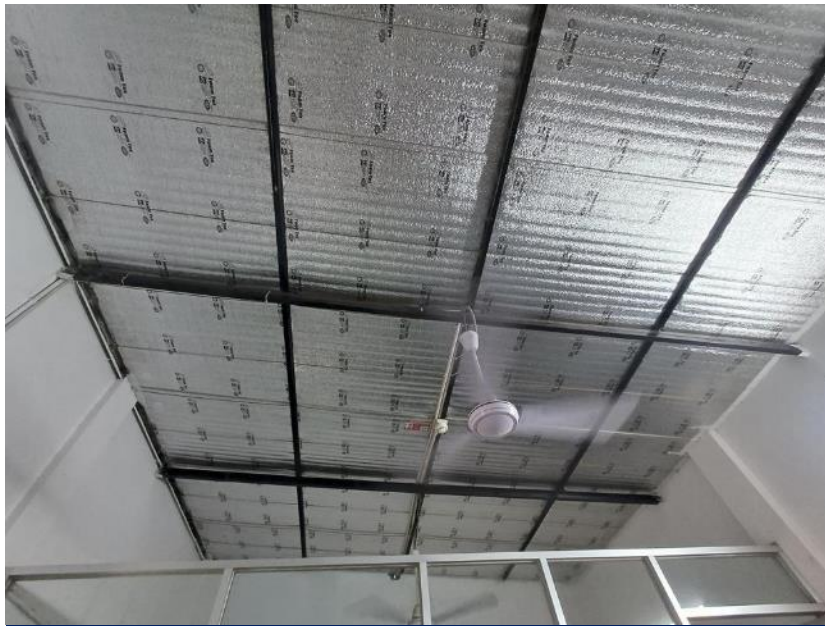
Framing of the structure
