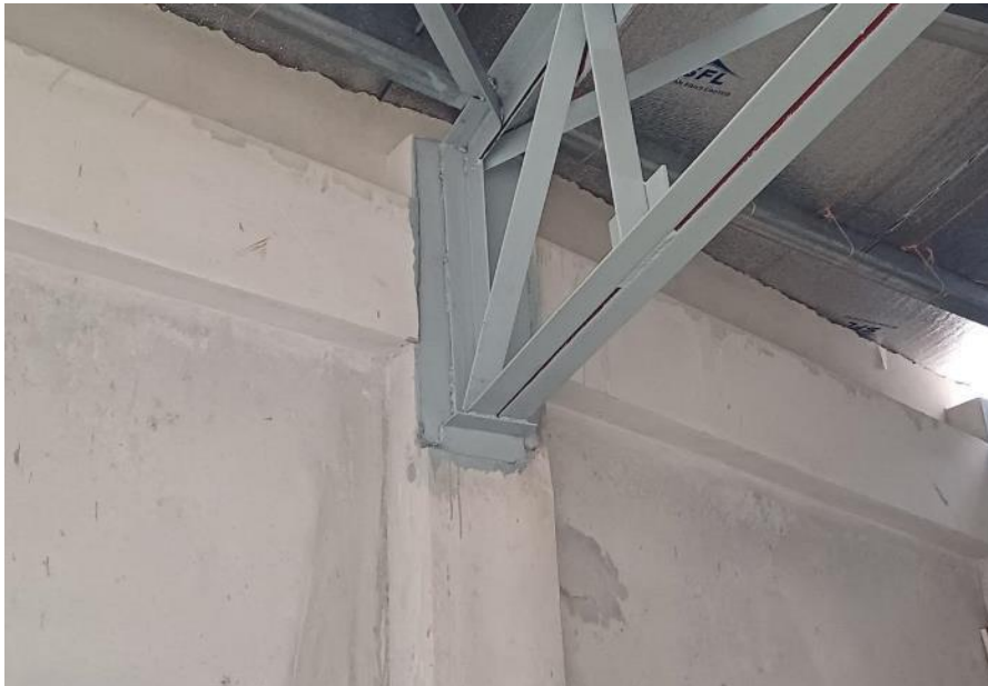
Truss connection with RC column
