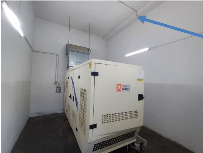
Beam on site
