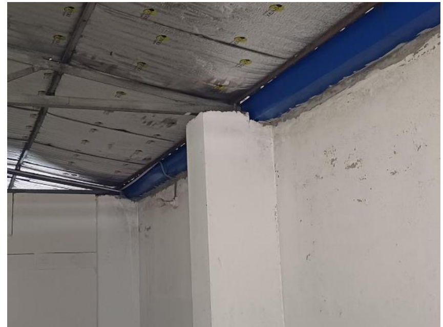
Truss frame connection with column
