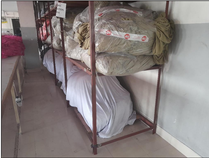
Storage racks were found not anchored
