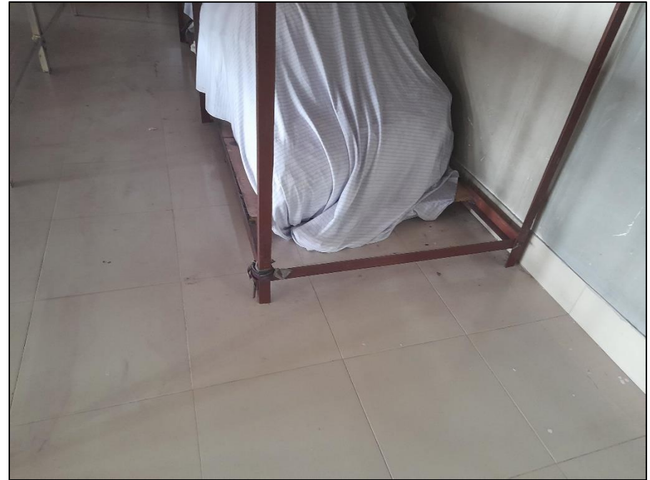
Storage racks were found not anchored
