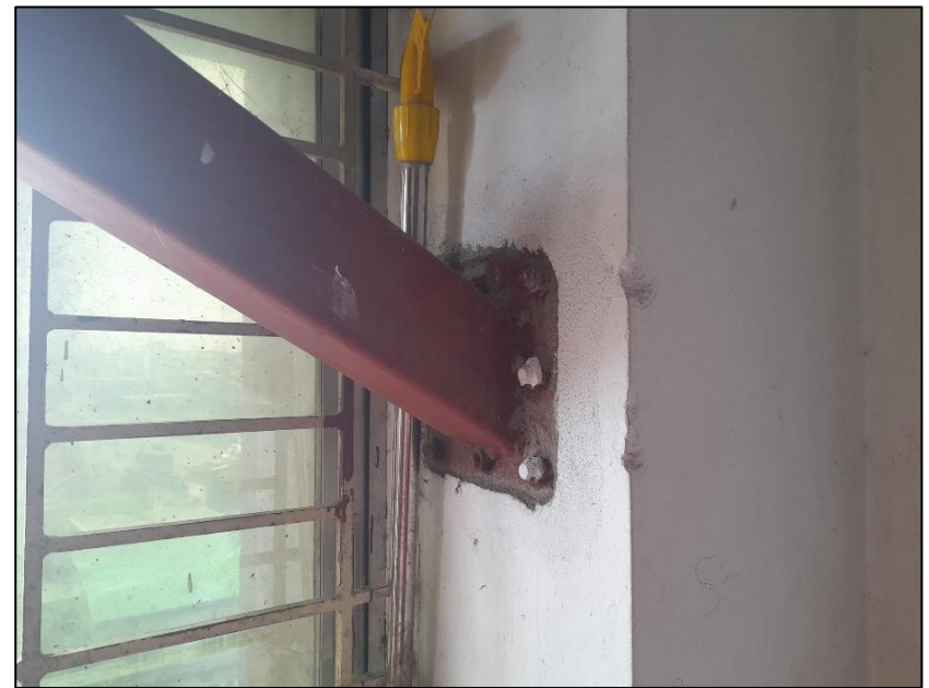
Retrofitted steel beam
