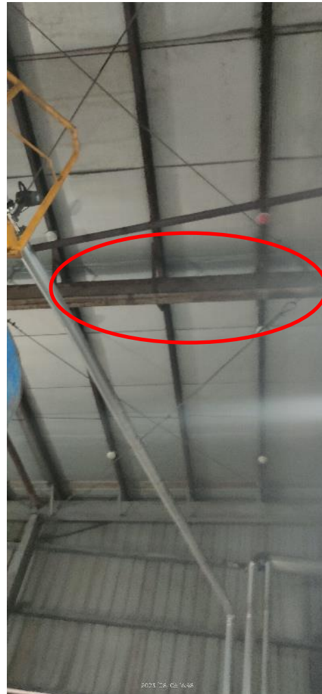
Corrosion in steel part of Building-3 (Boiler Building)
