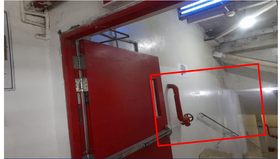
Wall bracing at Grid-1-E~F near to 3 rd floor stair not found during the inspection.
