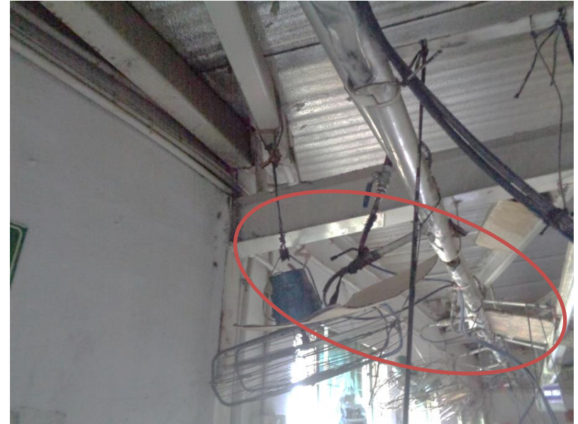
Missing compression strut along long direction
