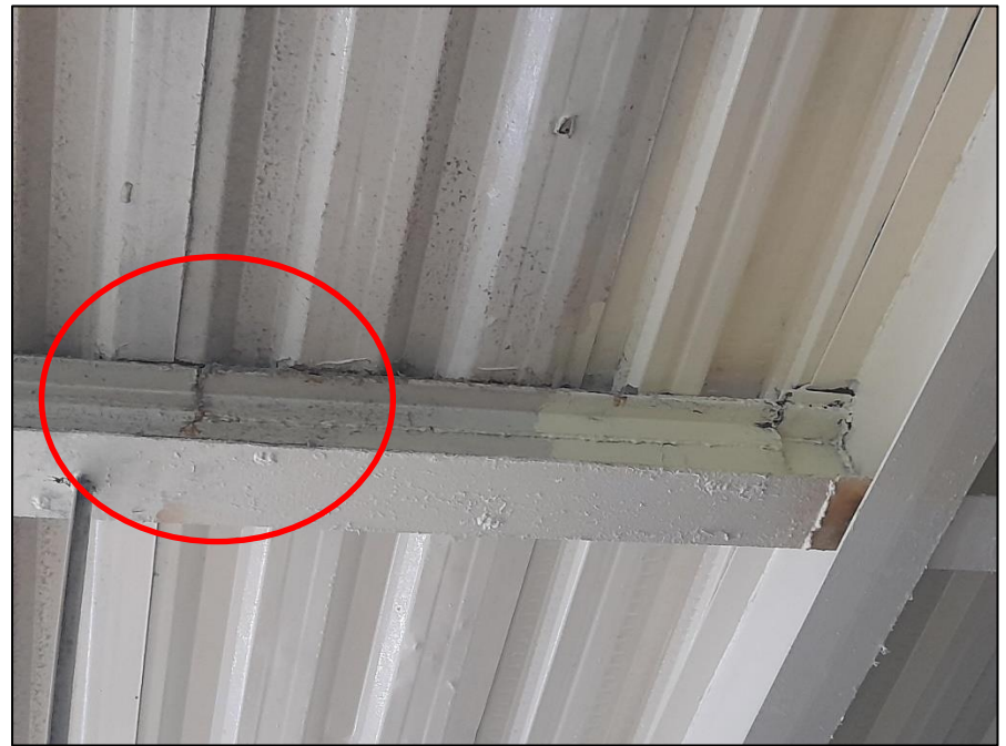
improper connections
