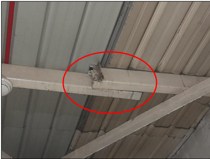
improper connections
