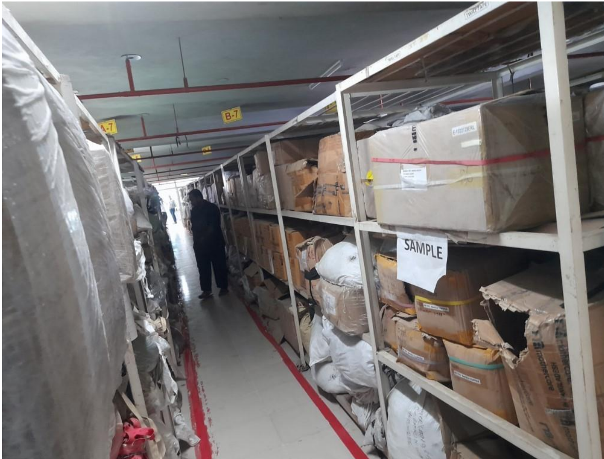
Storage rack found within the building without braced/anchored
