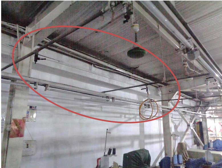
Missing compression strut along long direction
