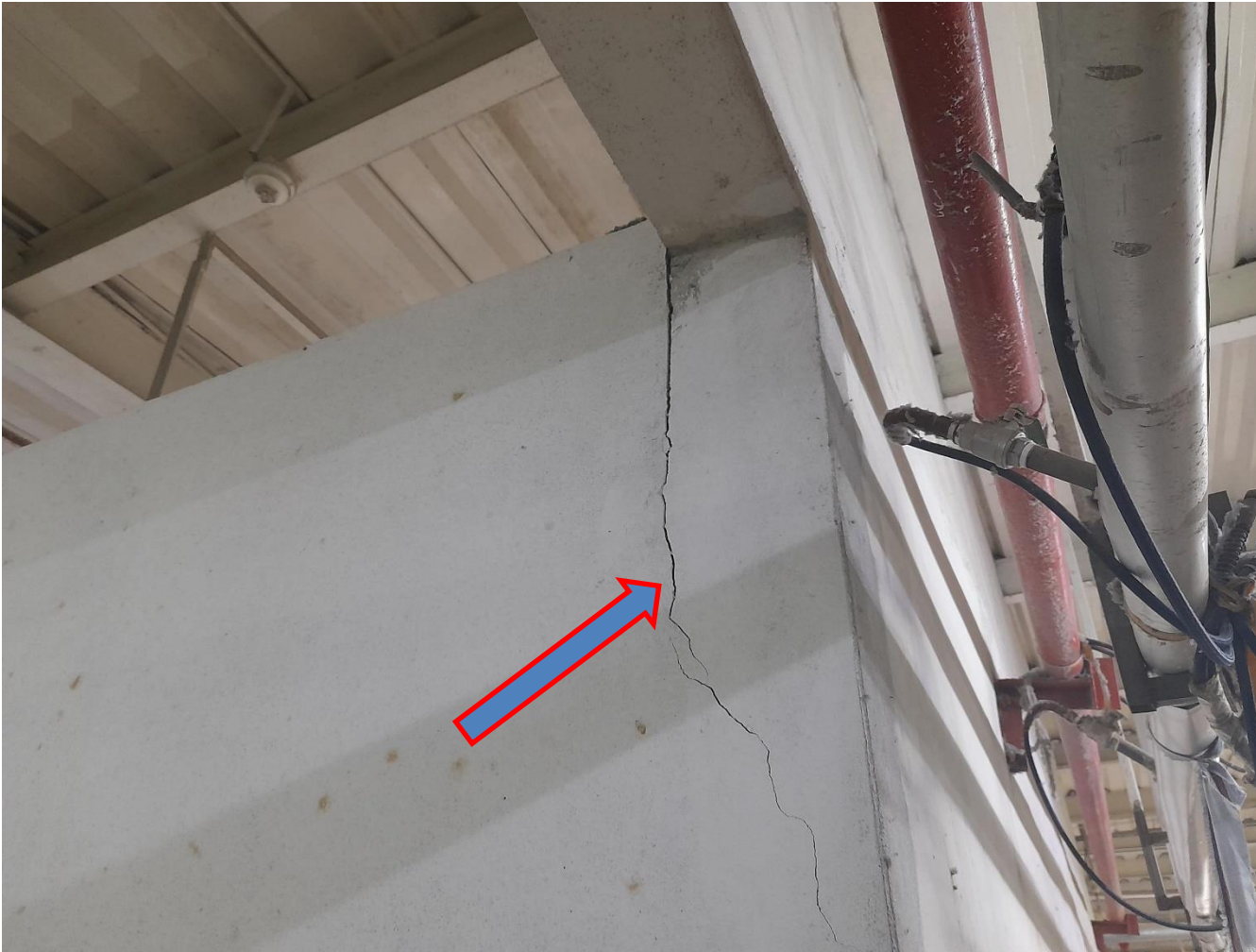
Crack in brick walls
