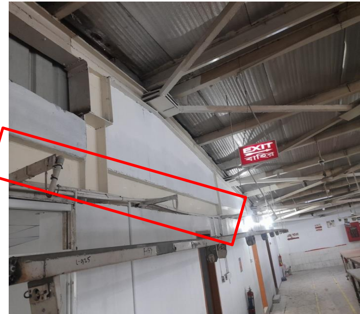
Beam of Grid-11: Not retrofitted
