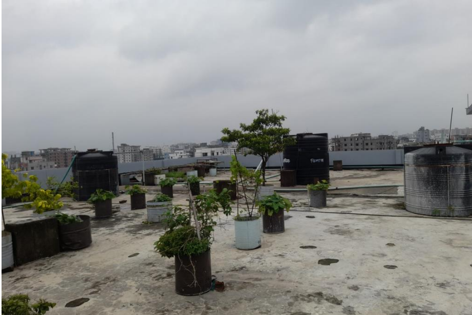
Two water tanks and gardening on the roof
