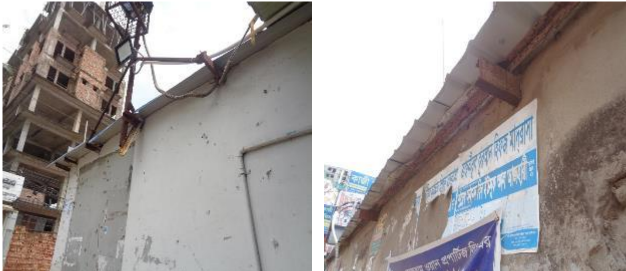
Connection of steel members and brick wall
