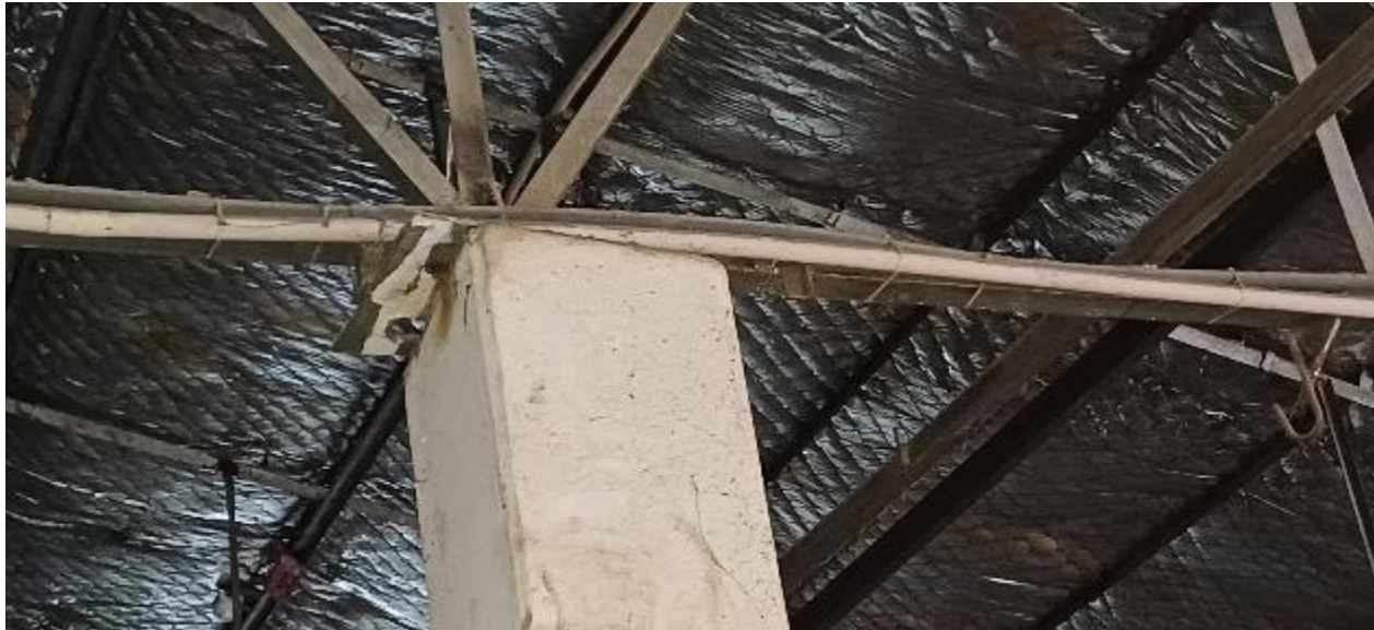
Connection of roof truss to RC column
