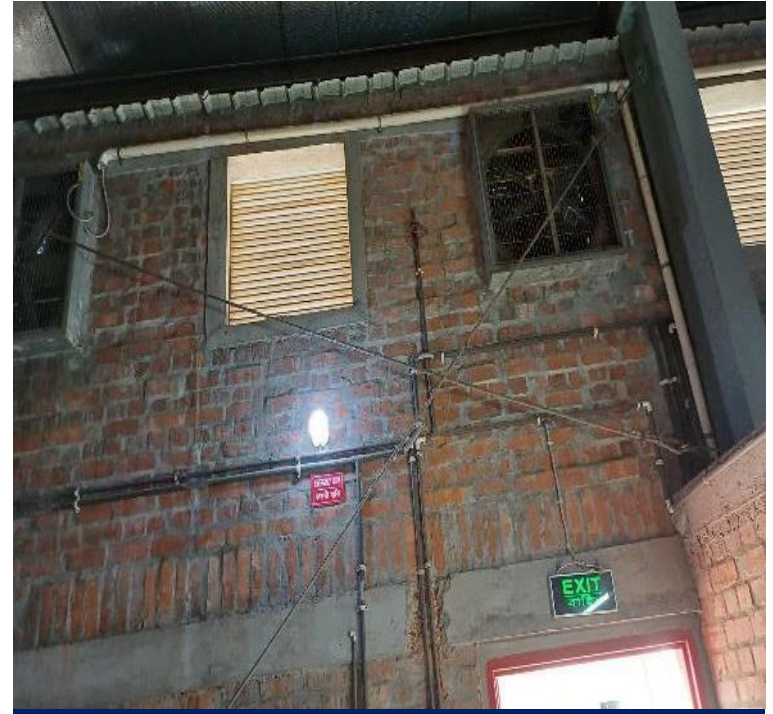
Eccentric vertical bracing
