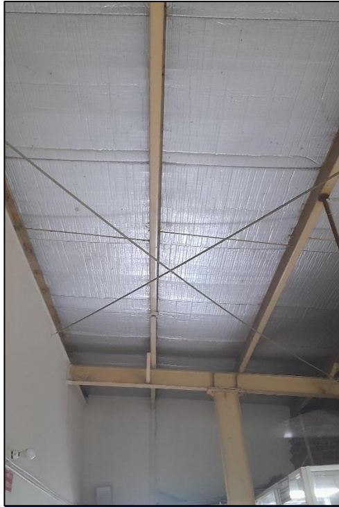
Roof & wall bracing provided
