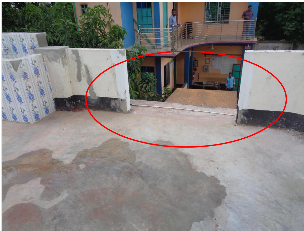
Opening at parapet wall
