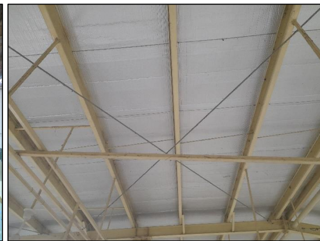
Roof bracing
