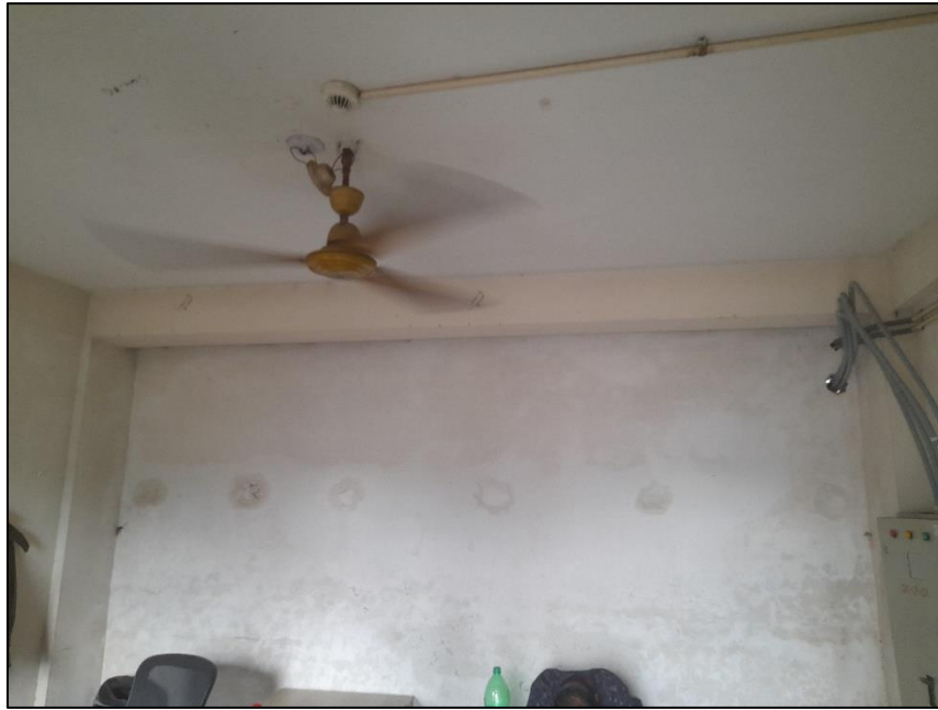
Inside of Security Guard Room
