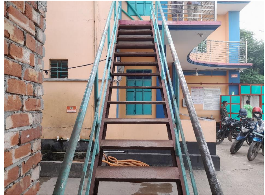
Non-engineered steel stair
