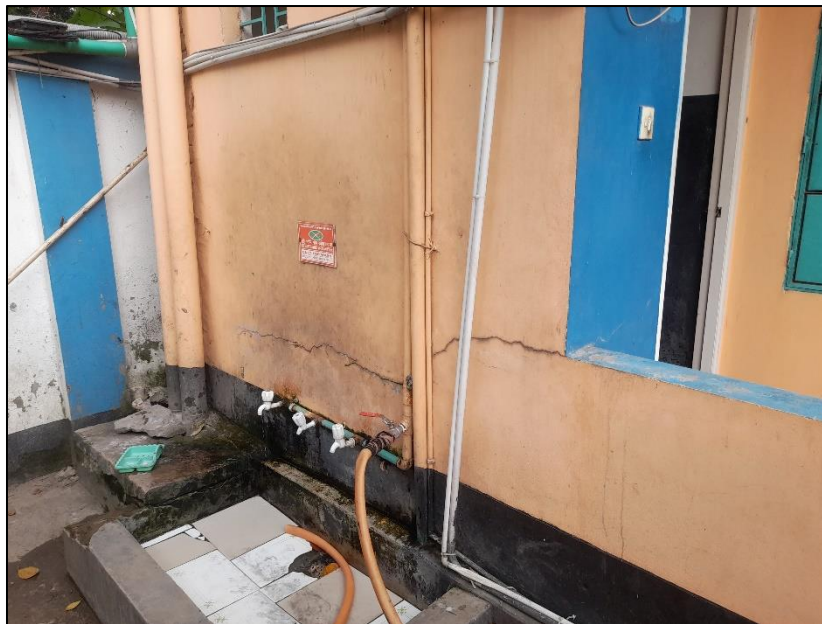
Cracks on masonry walls
