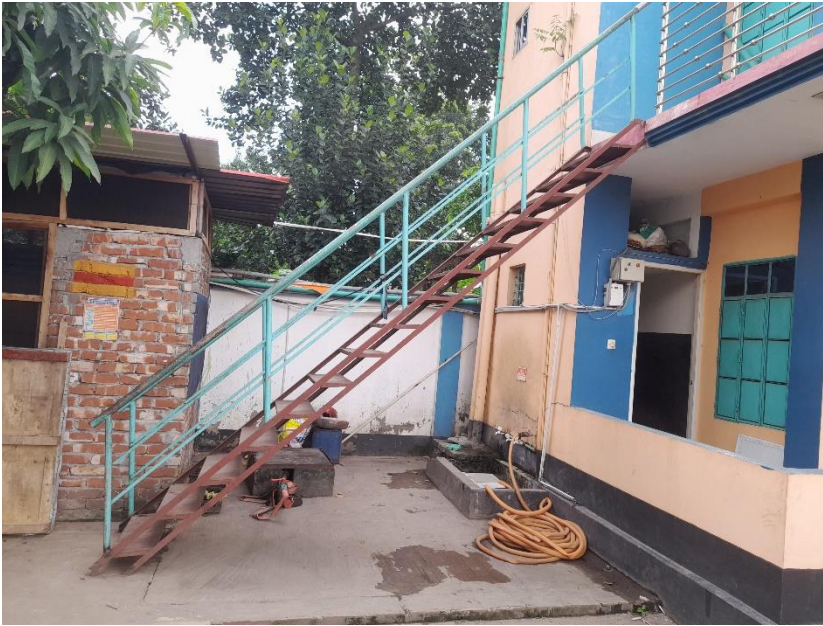
Non-engineered steel stair
