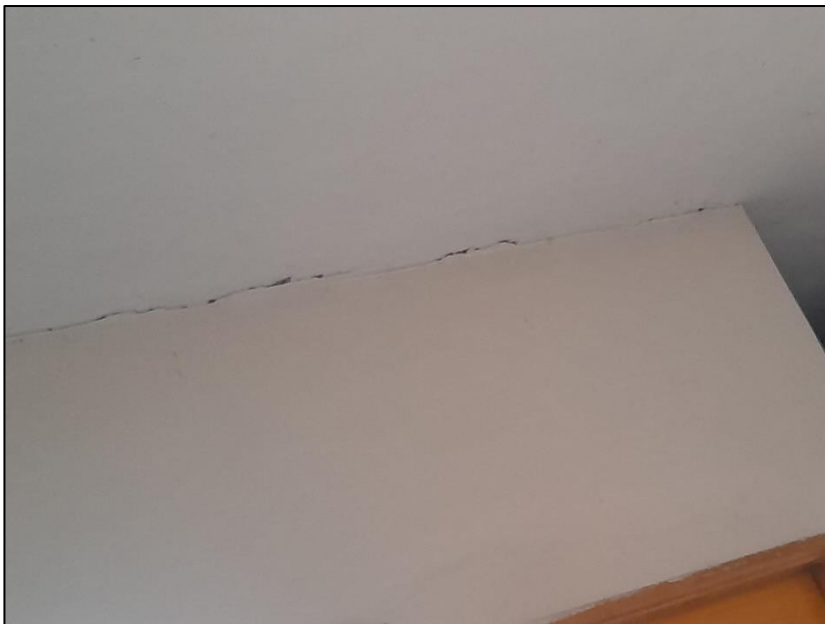
Cracks on masonry walls
