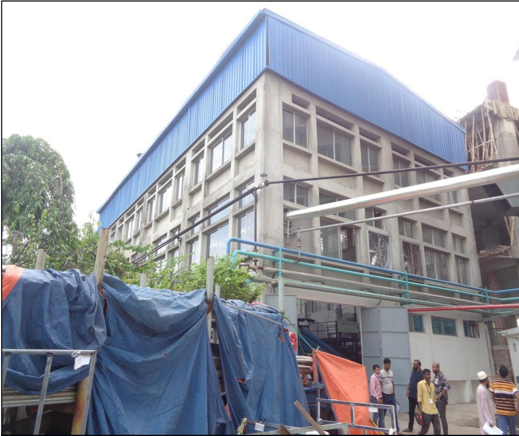
Jhut Boiler Shed
