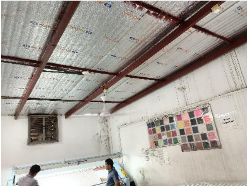
Fabric Inspection Room
