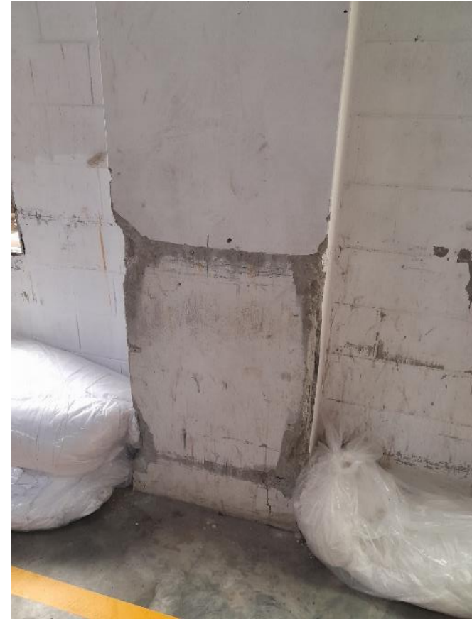
Damage RC column due to trolley Impact
