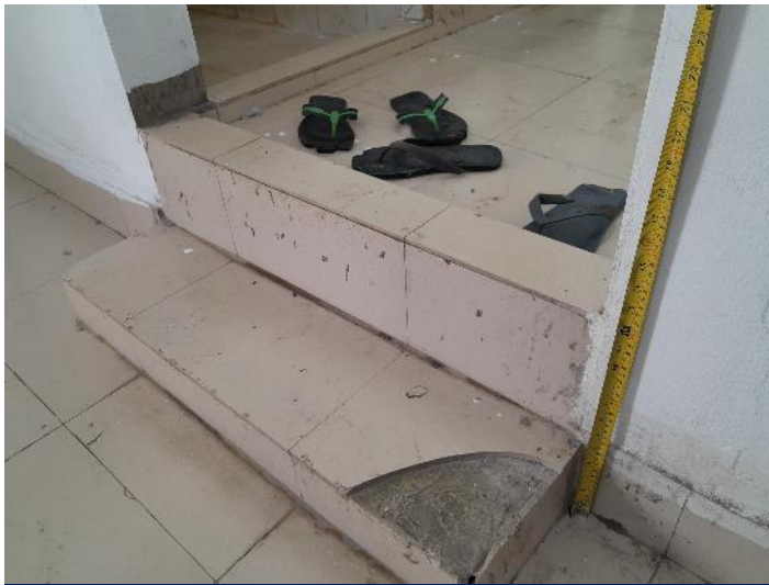
Onsite toilet build-up
