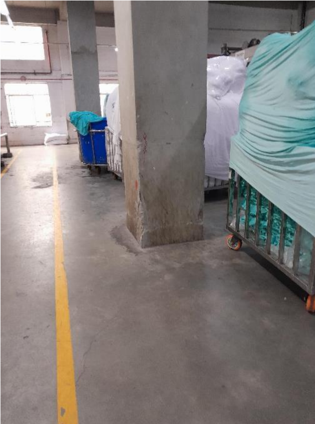
Damage RC column due to trolley Impact
