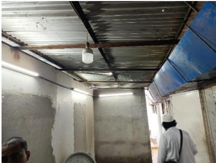
Shed-09 (Dining Shed)
