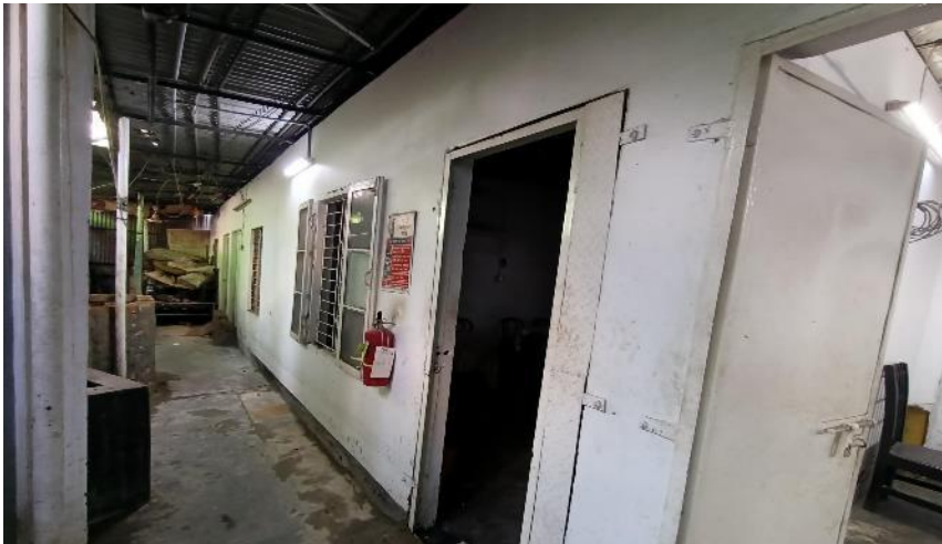
Shed-09 (Dining Shed)
