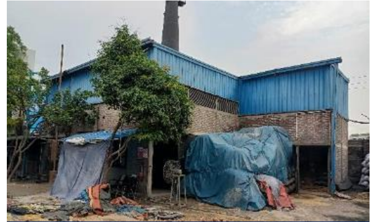
Shed-04 (Husk Boiler)
