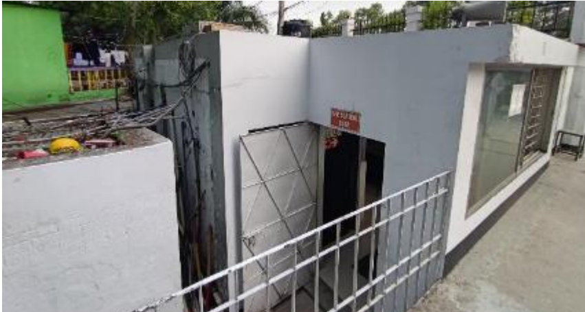
Building-06 (Guard Room)
