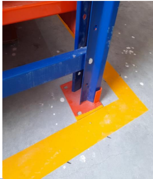
Racks and plastic water tanks not anchored or braced
