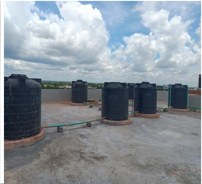
Racks and plastic water tanks not anchored or braced
