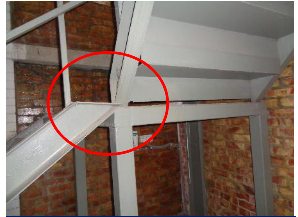
Less contact surface of connection
