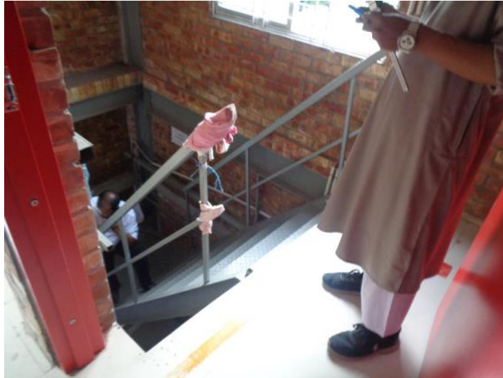
Falling hazard from stair landing
