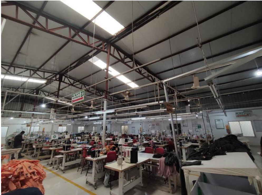
No load transfer media & bracings at roof
