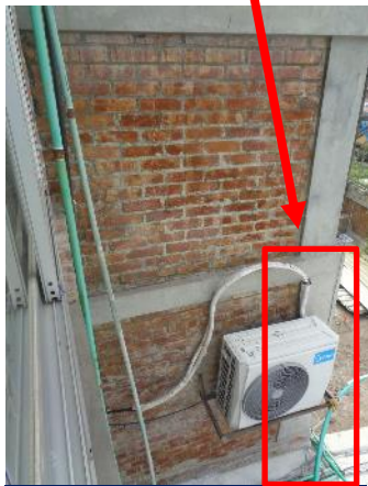
Column built up-to ground floor roof
