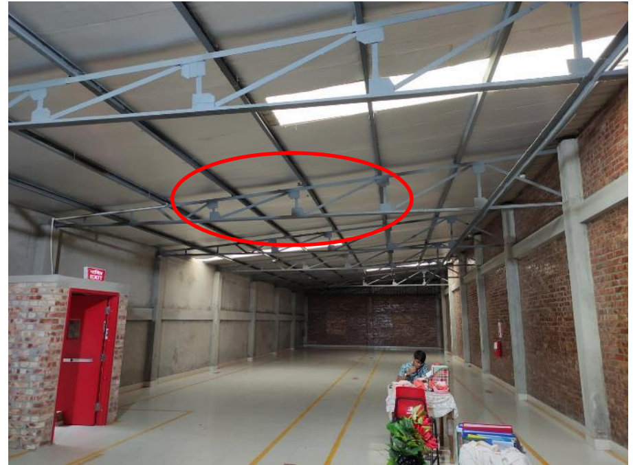
Truss angle direction (on-site condition)
