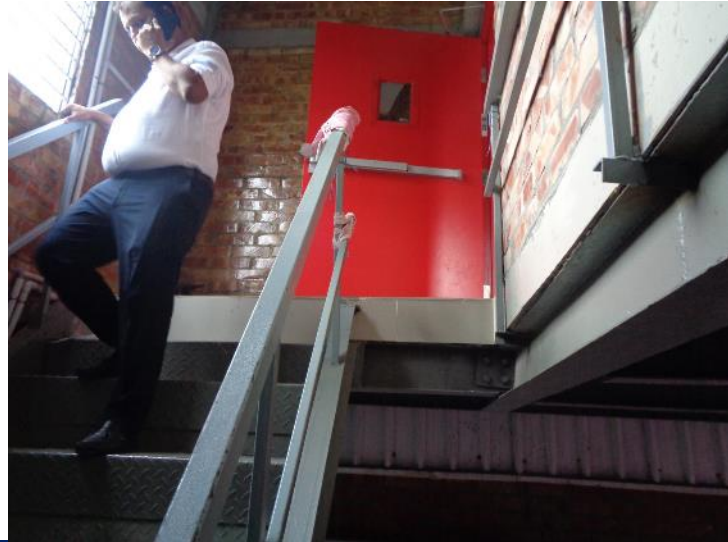
Falling hazard from stair landing
