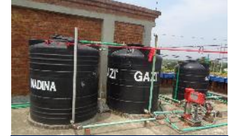
Source of Loads: Brick walls and water tanks
