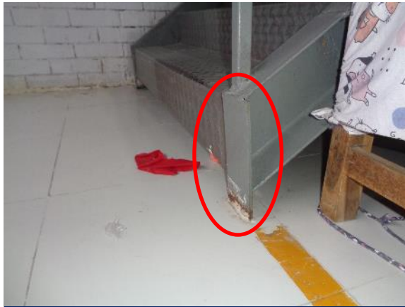
Stair rested on a thin plate leg
