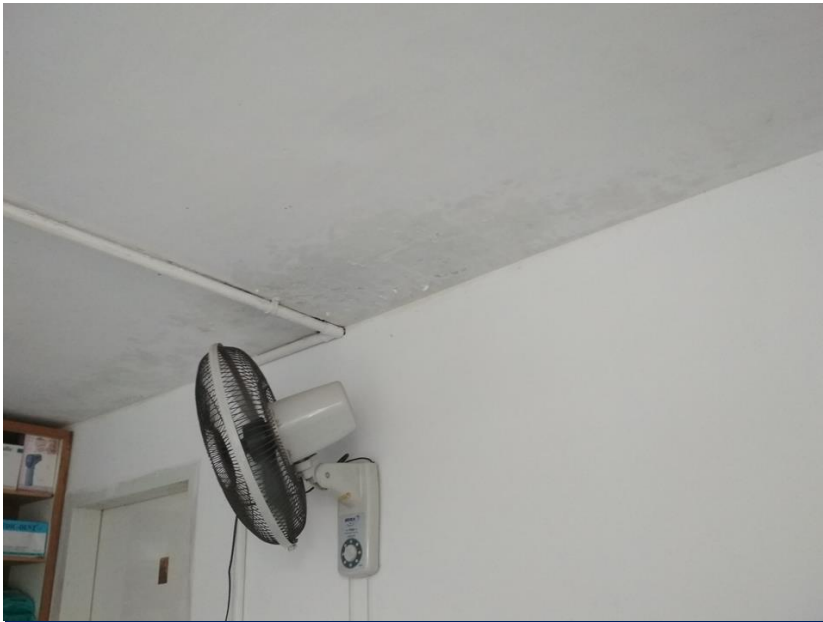
Dampness on roof slab
