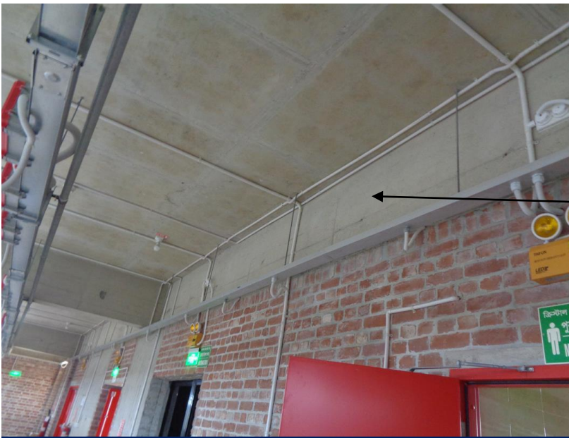
Beam on site: 900 mm depth
