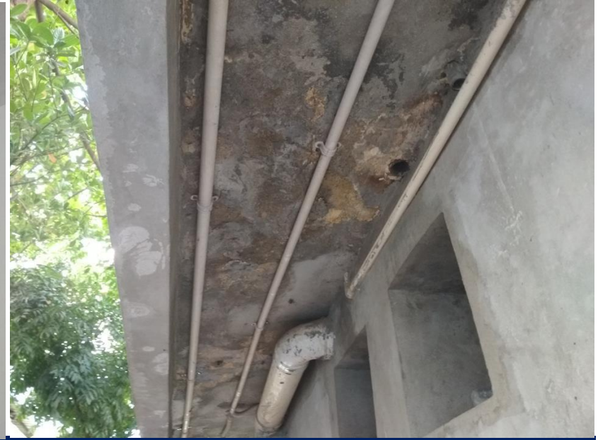
Dampness on roof slab
