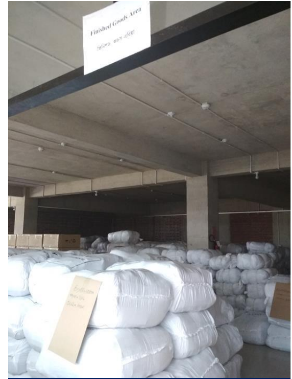
Heavy storage on suspended ground floor
