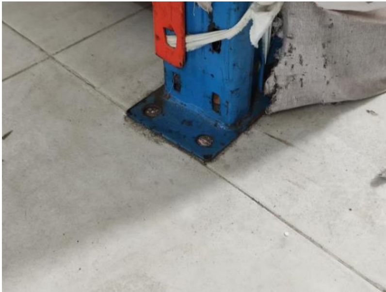
Lack of anchorage of storage rack
