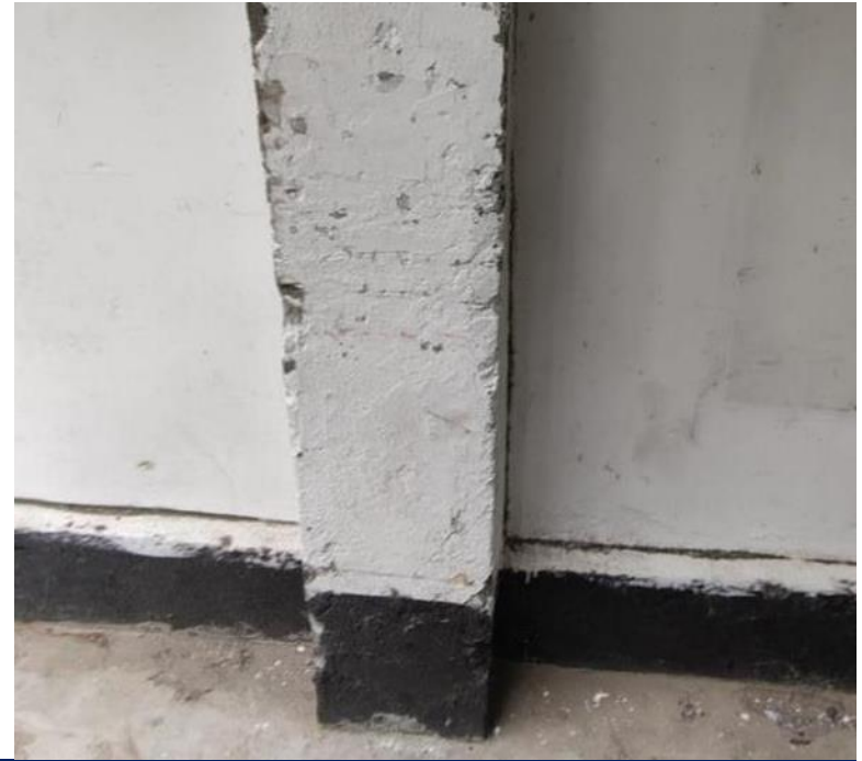
Damage RC Column due to trolley Impact
