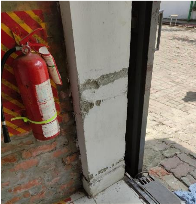
Damage RC Column due to trolley Impact
