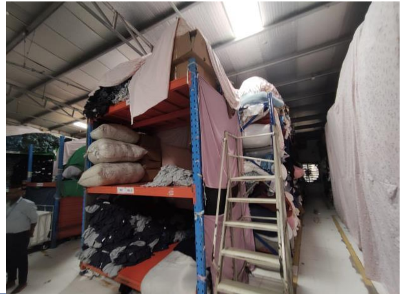
Lack of anchorage of storage rack
