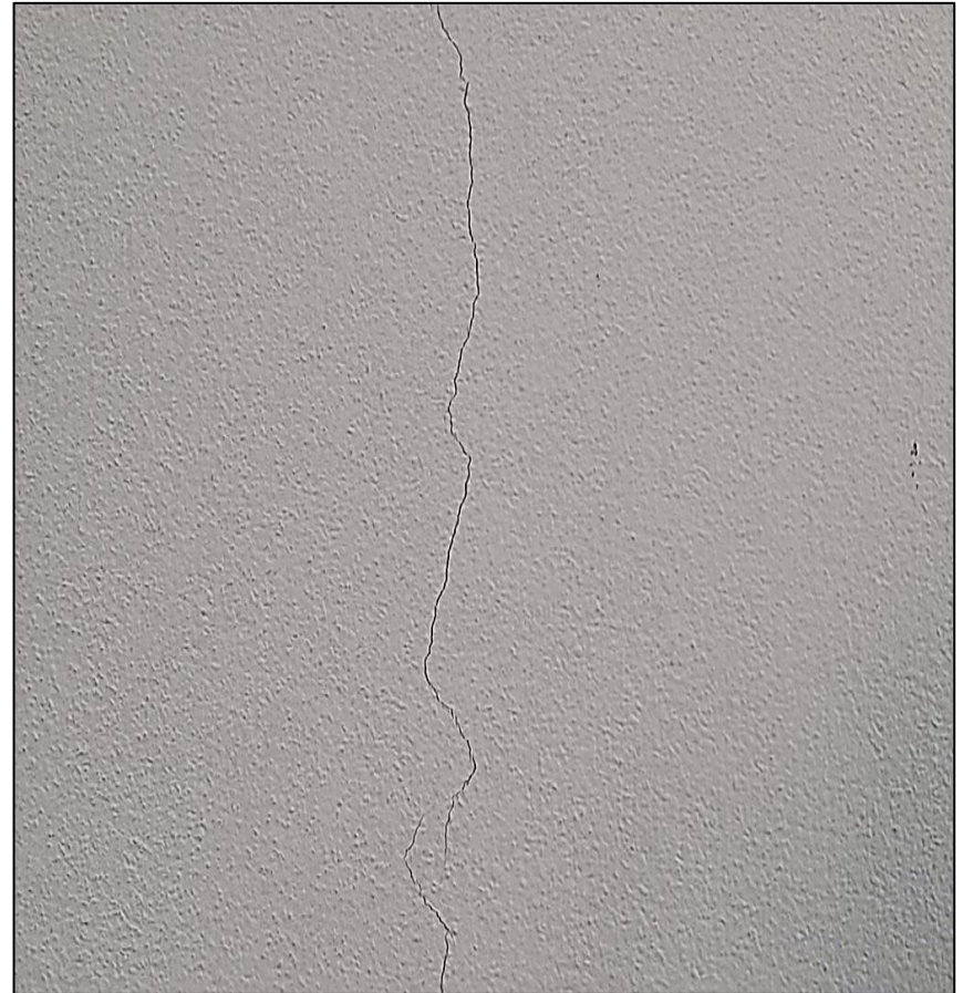
Brick Wall Crack
