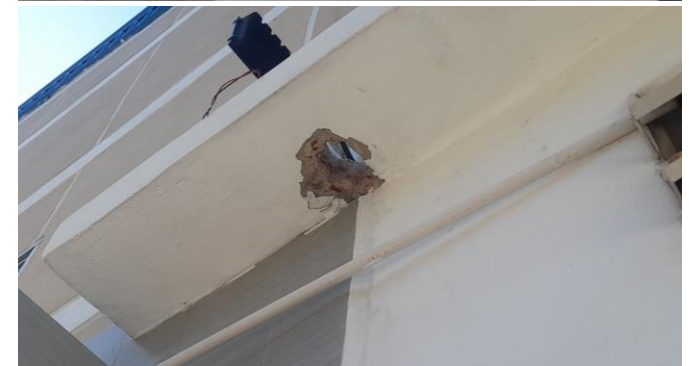
Compression Room Roof
