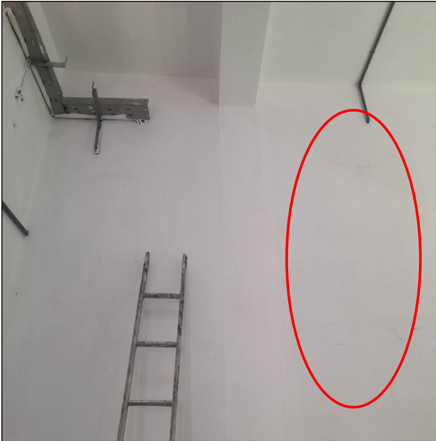
Brick Wall Crack
