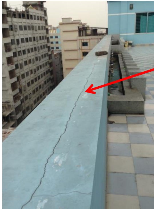
Parapet wall on west side (rear of building)
