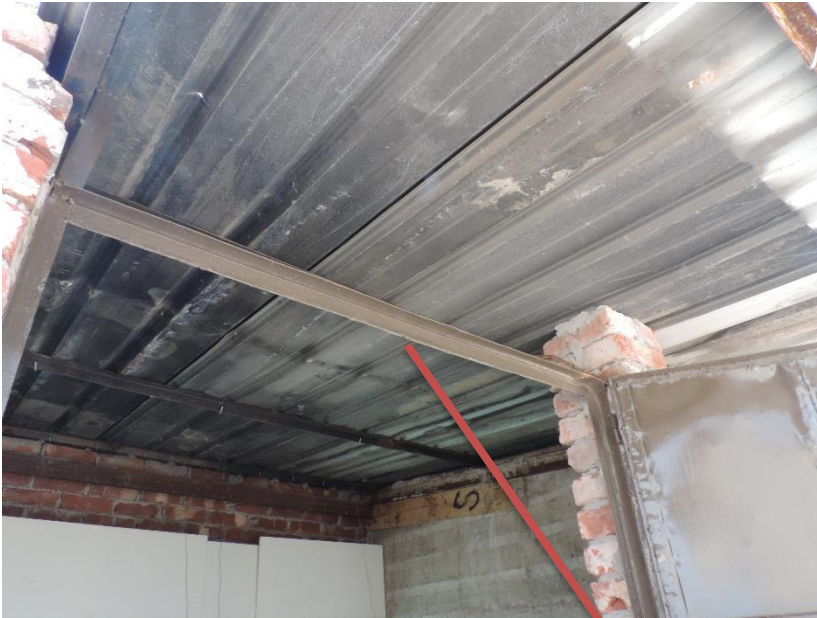
Non Engineered steel roof to stair core
