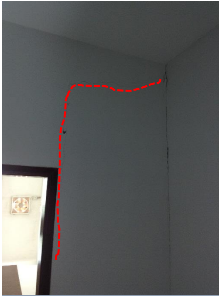
Minor cracks on walls perpendicular to cantilever on 5th floor
