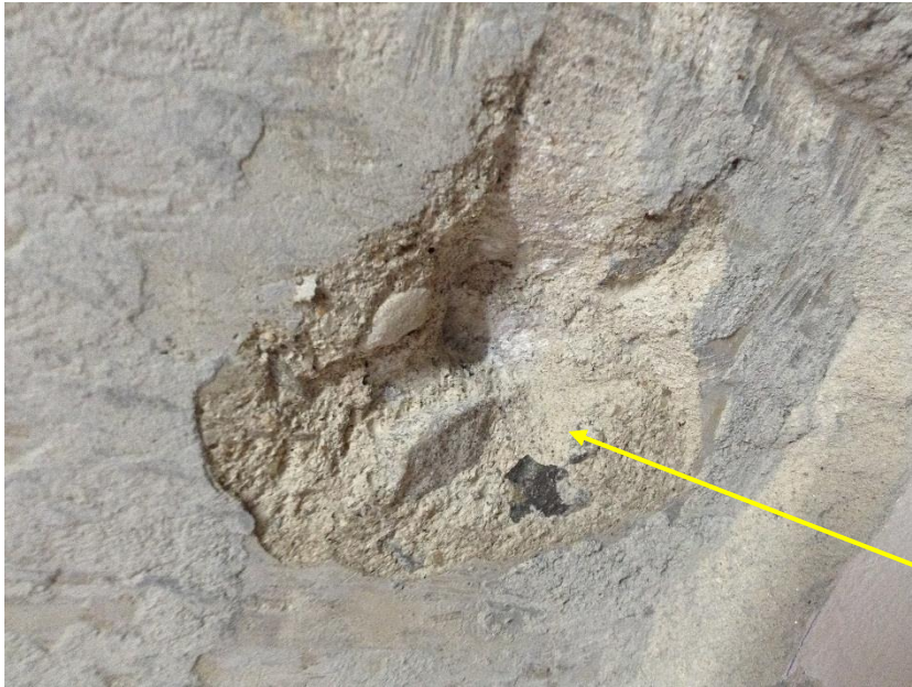
Stone Aggregate noted in ground floor columns
