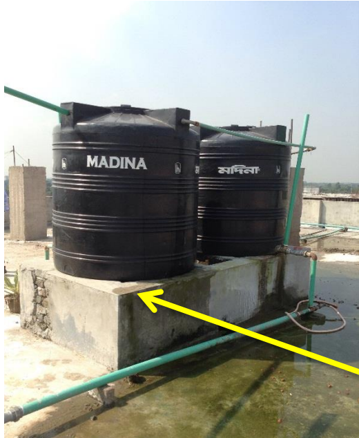
Water tank on roof. Capacity 2 x 2000L
