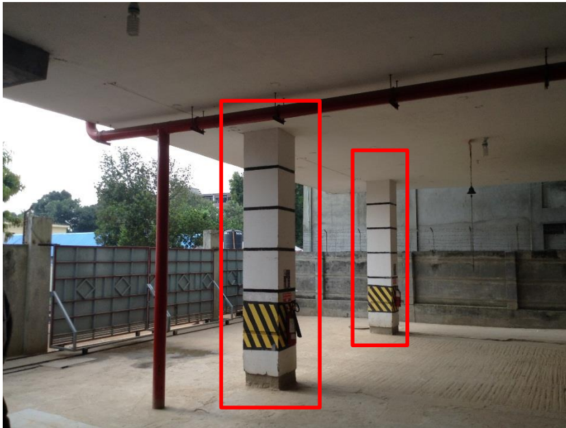
Columns in loading bay unprotected from traffic impact.
