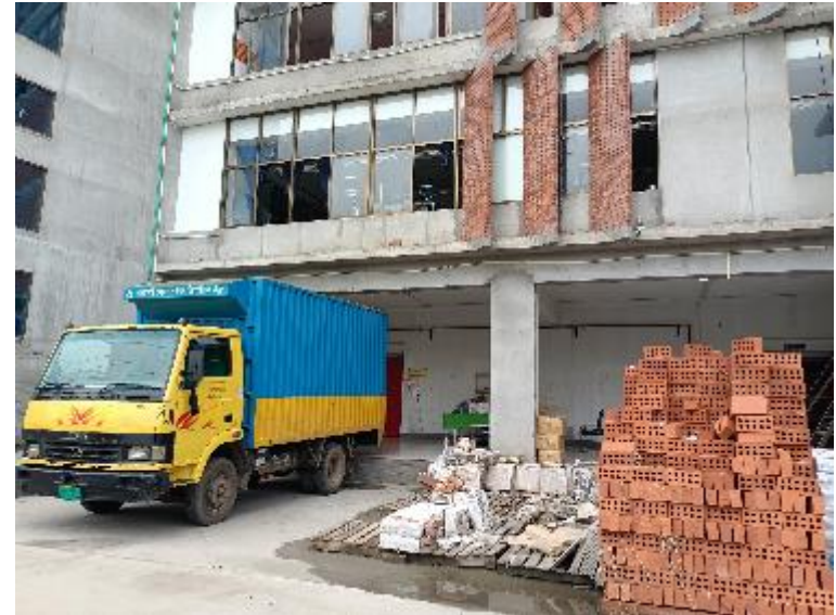
Column susceptible to vehicle impact
