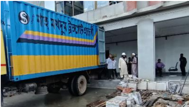
Beams adjacent to the driveway of loading unloading zone
