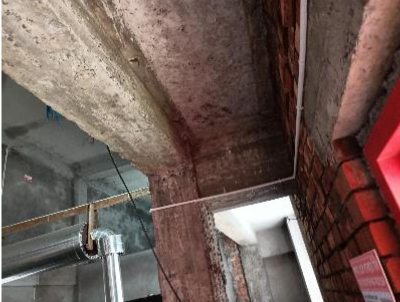
Additional slab at front
