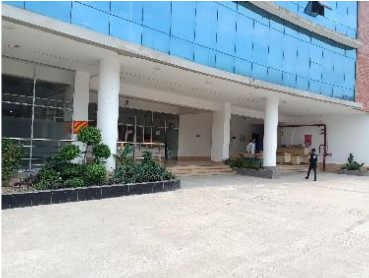
Column susceptible to vehicle impact
