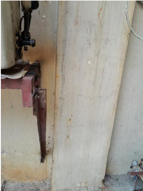
Corrosion crack observed in periphery columns
