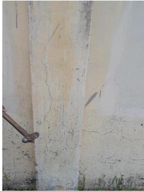
Corrosion crack observed in periphery columns
