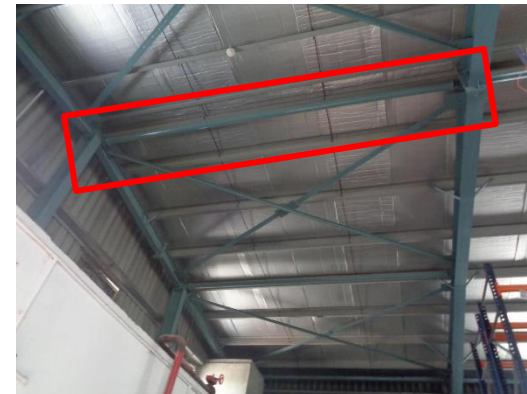
Compression strut layout drawing: I shaped strut (T1) at eave, ridge and end & central bays
