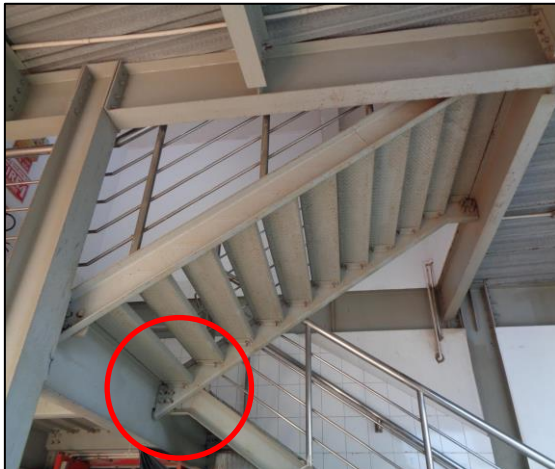
Oversized hole in bolted connection
