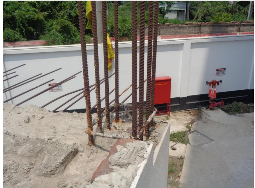
Exposed rebar on the roof which is prone to corrosion
