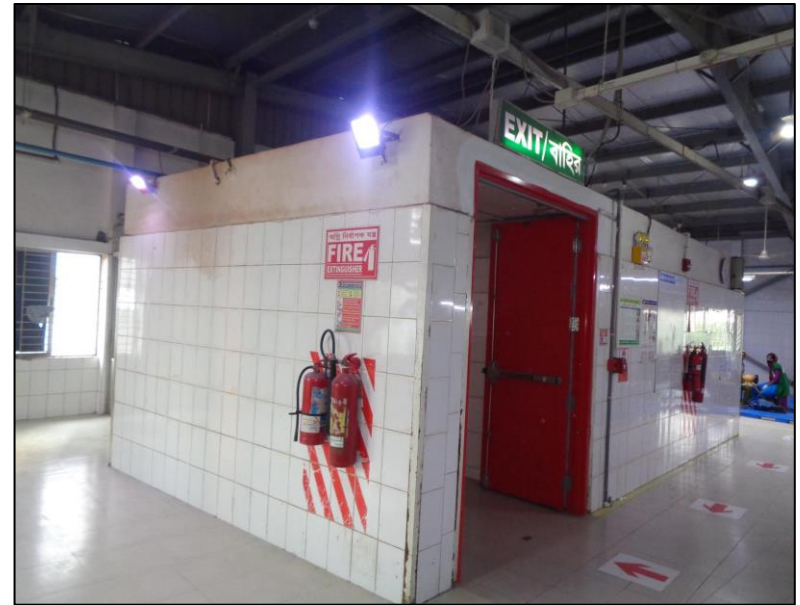
Undocumented 250mm masonry wall
