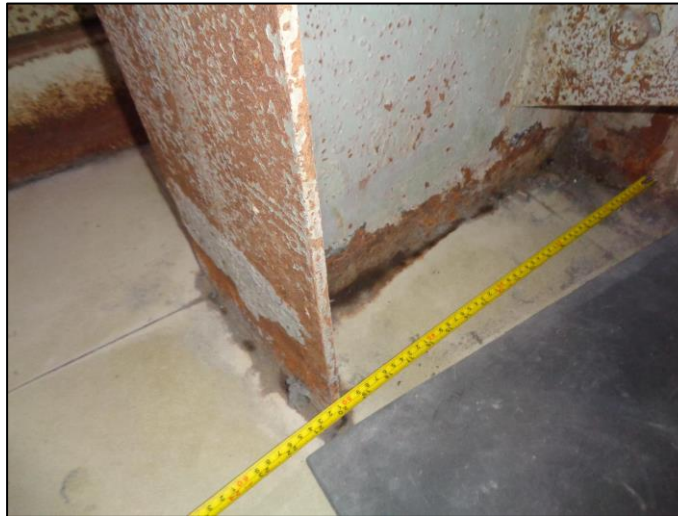
Corrosion in steel members
