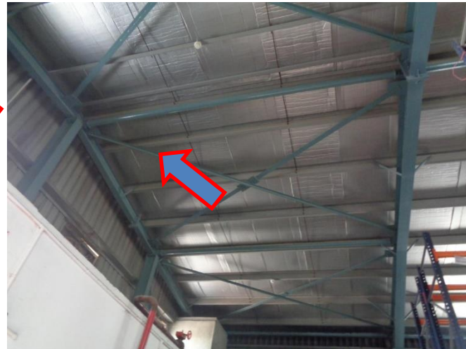
2L-50x50 mm bracing measured at roof
