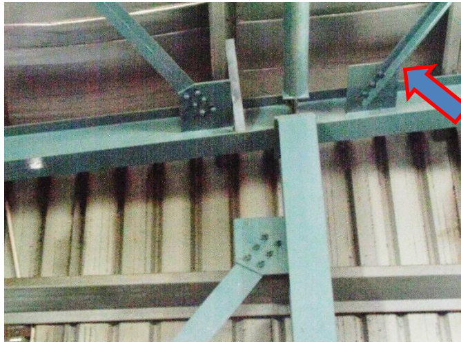
2L-50x50 mm bracing measured at roof
