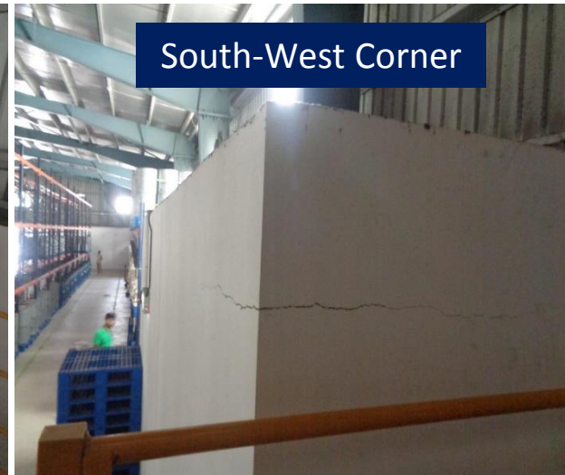
Crack in brick walls
