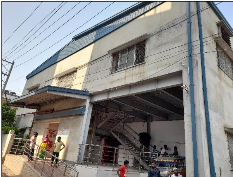
PP Spray Shed
