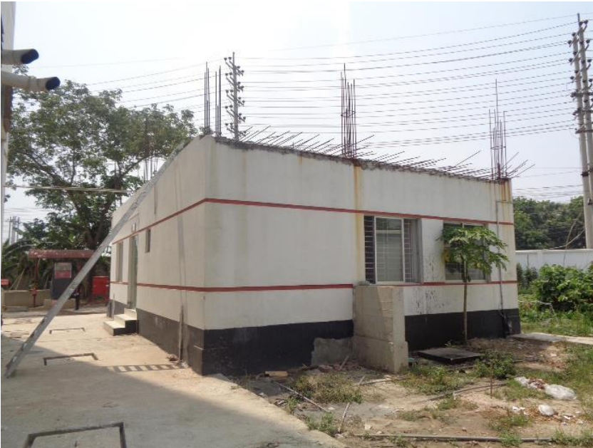
Exposed rebar on the roof which is prone to corrosion
