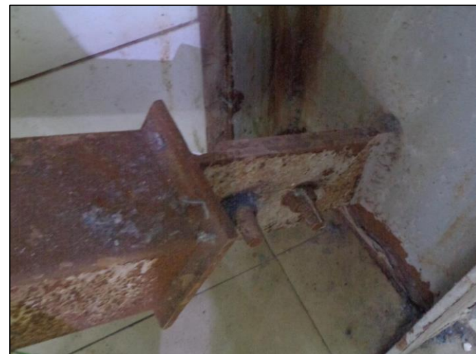
Corrosion in steel members
