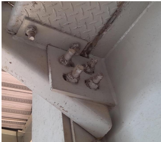
Oversized hole in bolted connection
