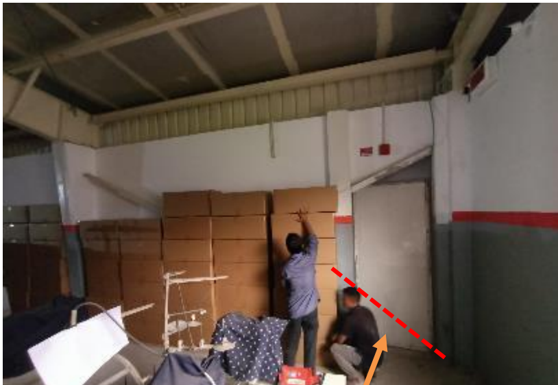
Missing bracing
