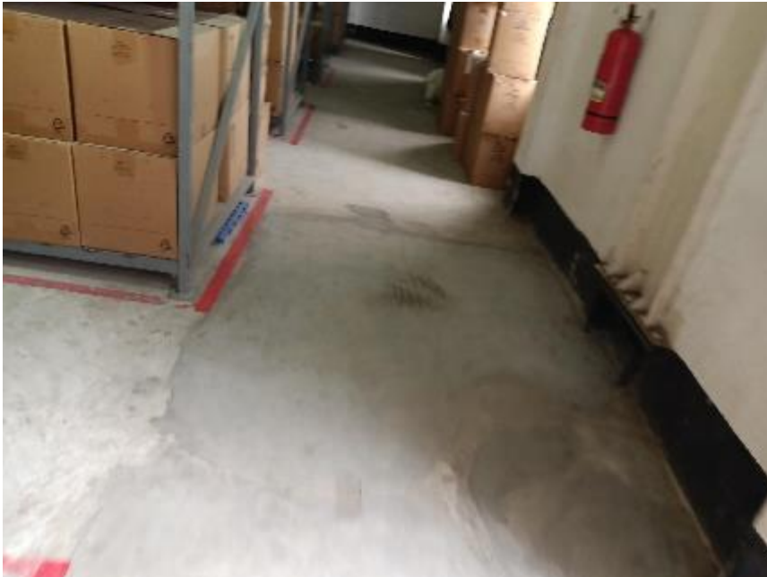
Non-anchored storage rack at several floors
