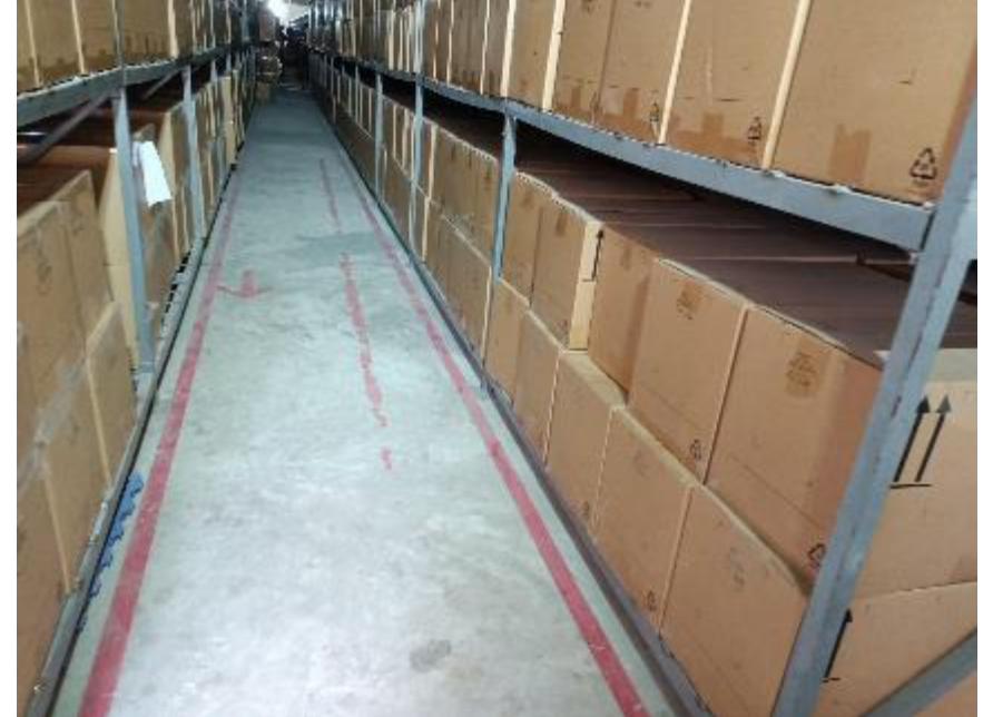
Non-anchored storage rack at several floors
