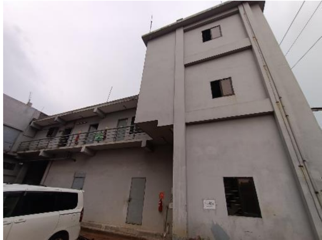
No design report was available for Utility Building
