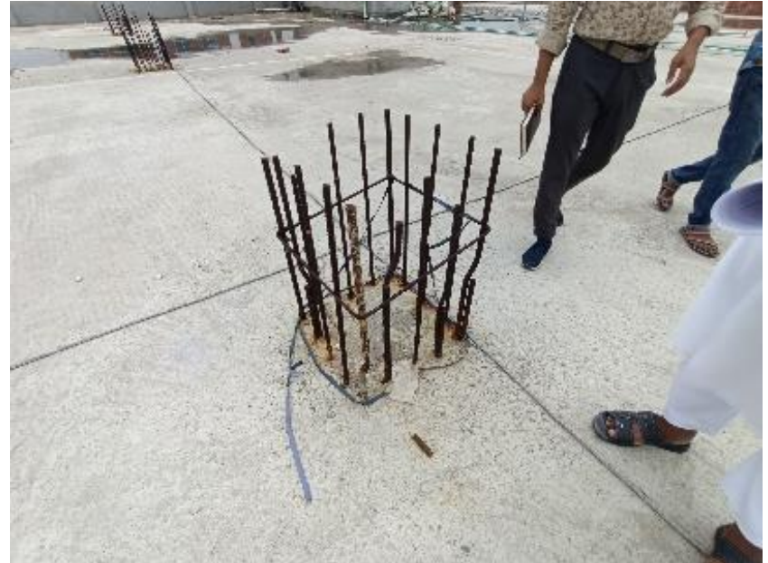
Exposed rebar at column on roof
