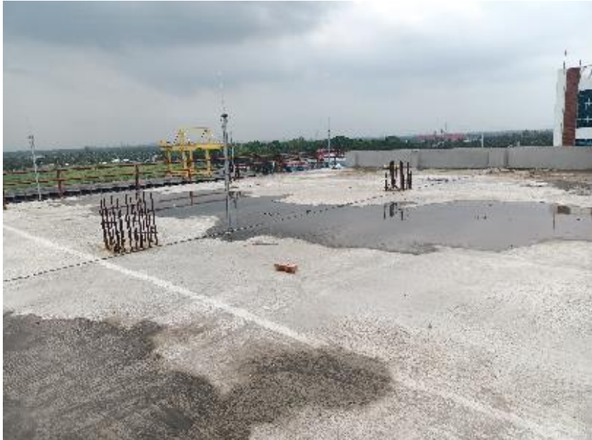
Exposed rebar at column on roof
