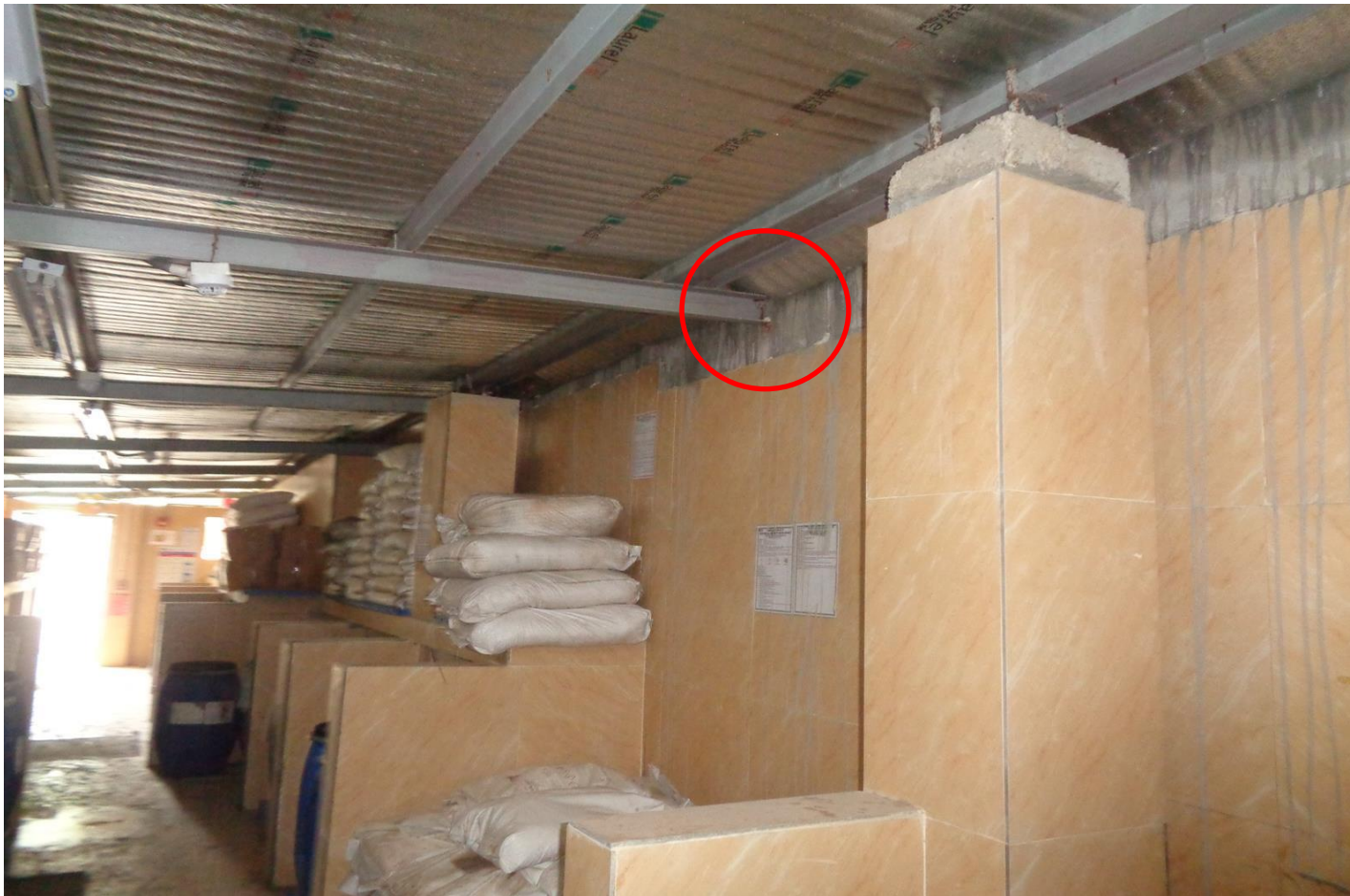
Rafter inserted to brick wall
