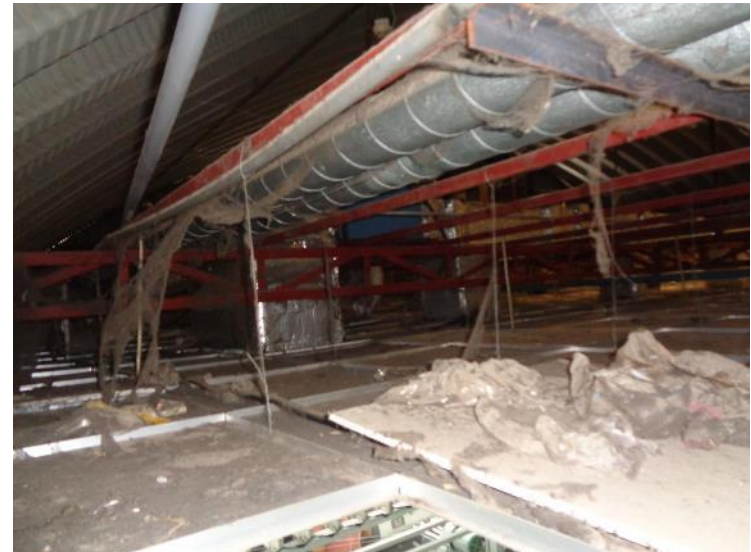
Individual truss-column frame for MEP
