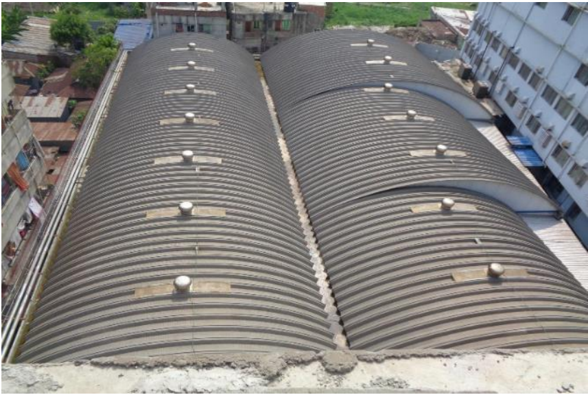
Metal curved roof decking system: No lateral support perpendicular to the deck rib
