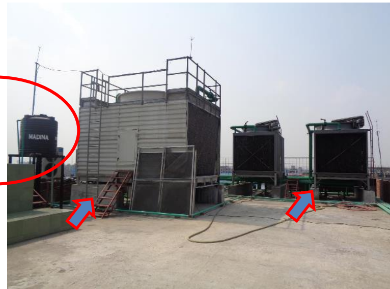
Floor built-ups and water tanks on the roof
