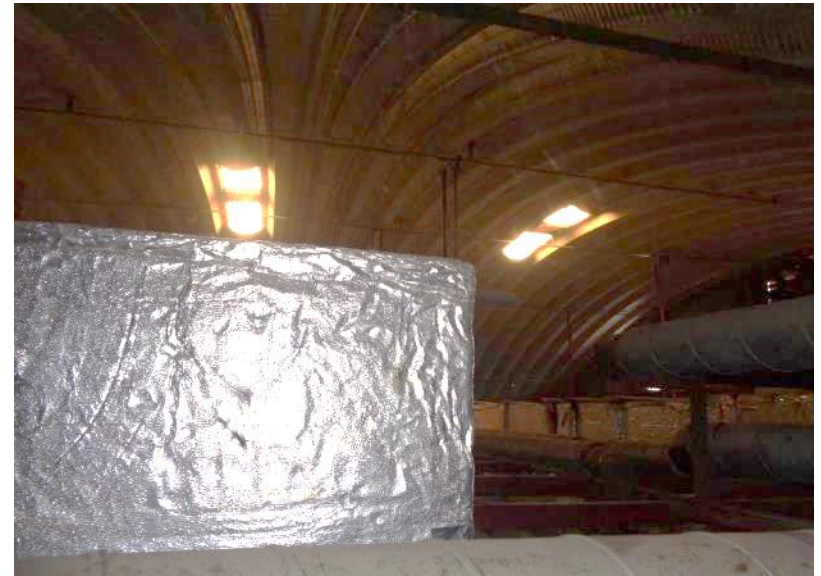
Metal curved roof decking system: No lateral support perpendicular to the deck rib
