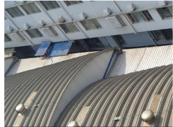
Roof extension on north
