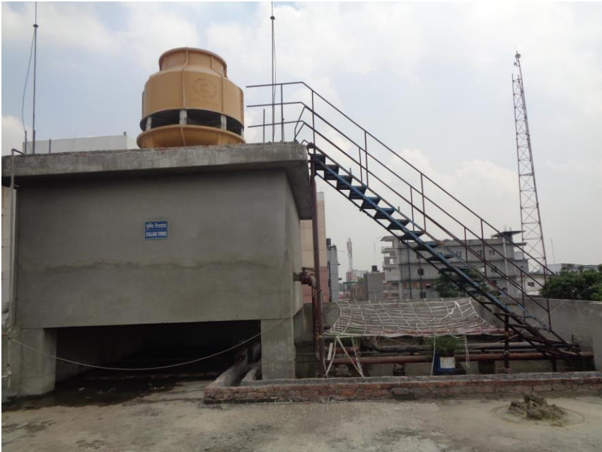
Inadequate and corroded steel ladder
