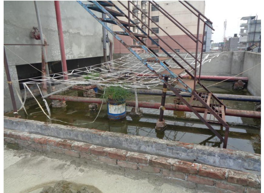
Inadequate and corroded steel ladder
