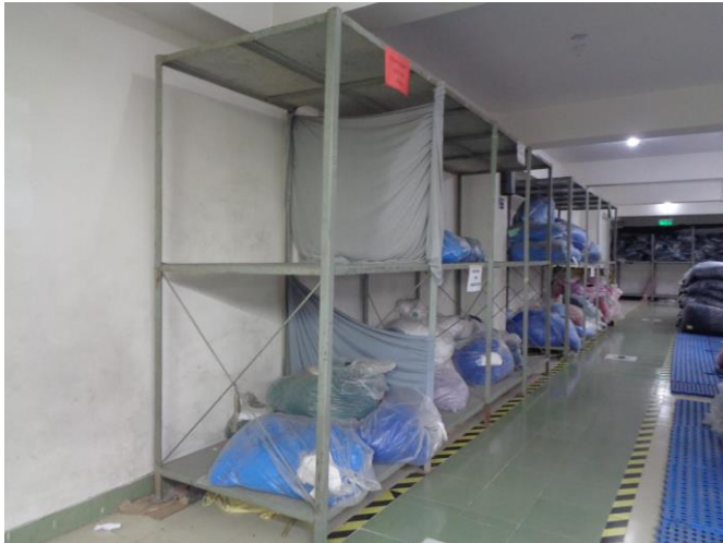
Lack of anchorage of storage racks and water tank
