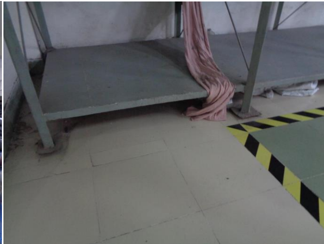
Lack of anchorage of storage racks and water tank
