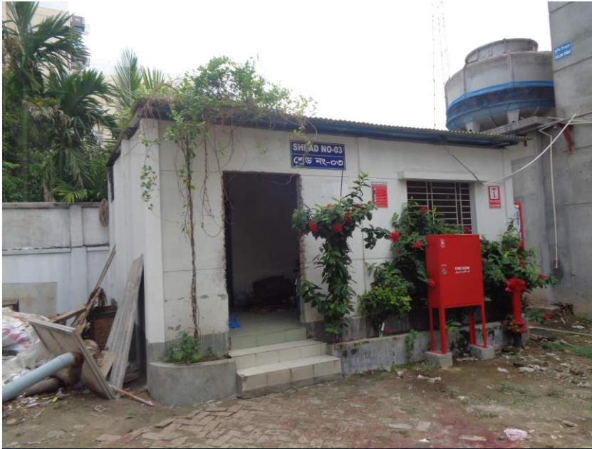
Lack of anchorage of steel roof
