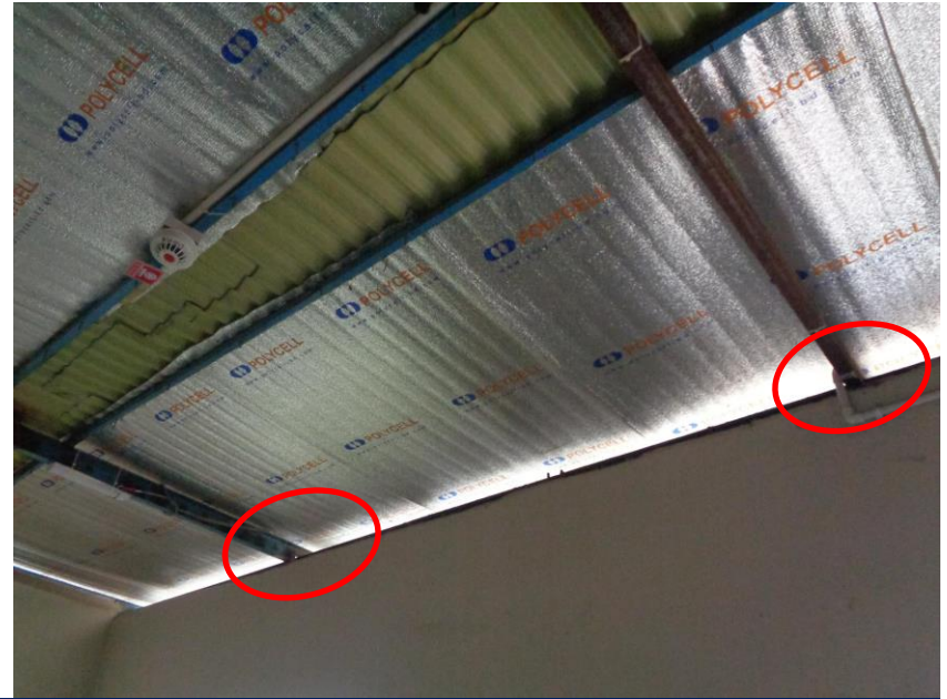
Lack of anchorage of steel roof
