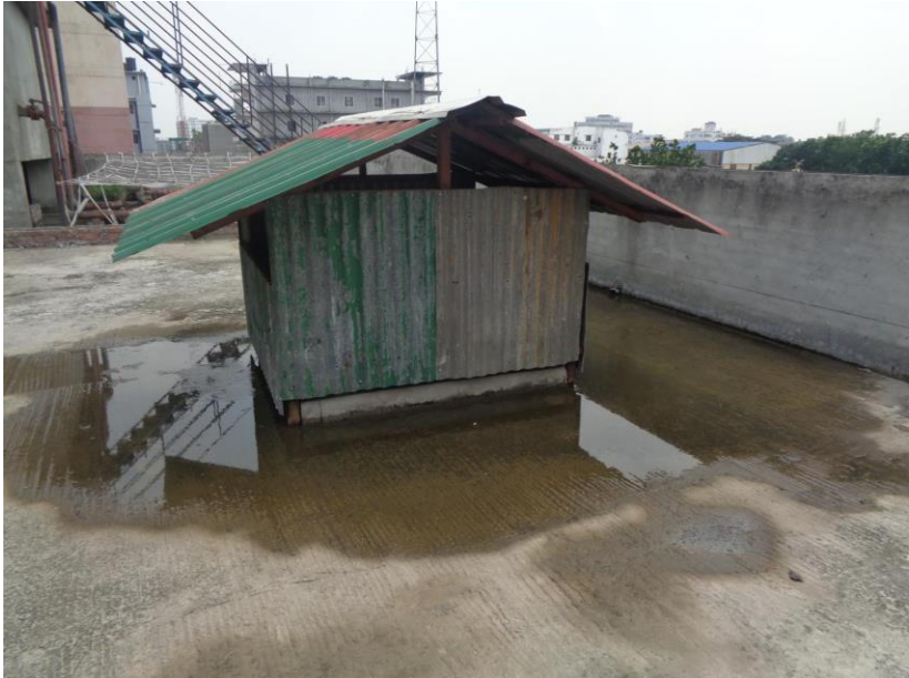
Water ponding on the roof
