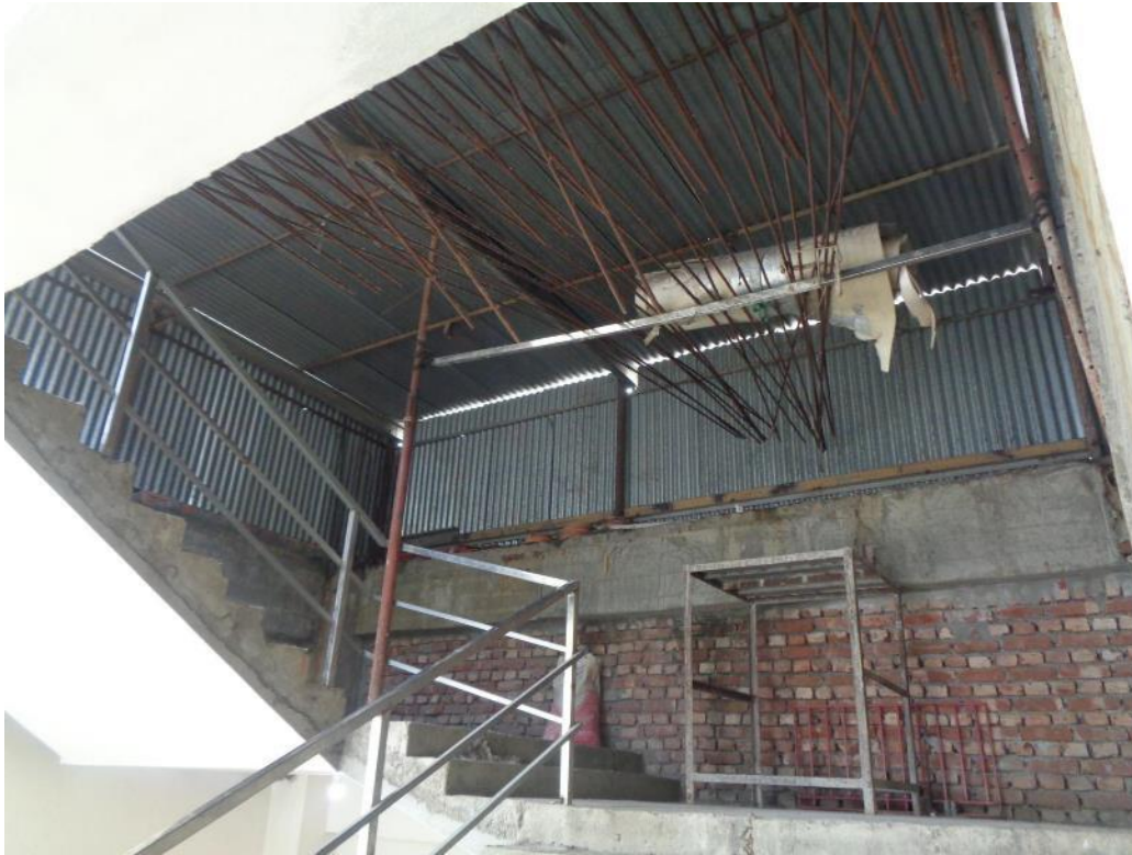
Non-engineered steel roof on the stair
