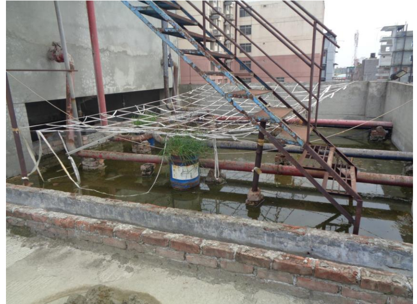
Water ponding on the roof
