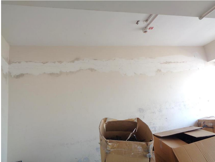
Crack on walls
