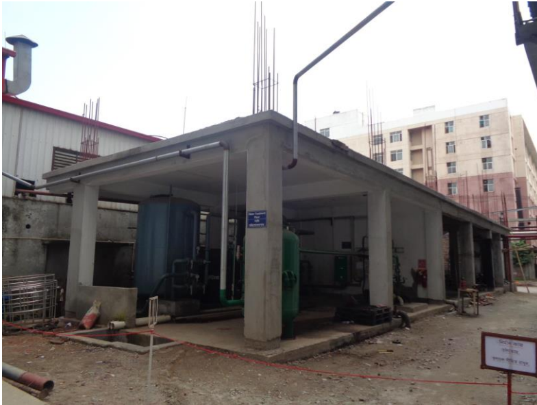
Lack of fall protection in the roof and open stair
