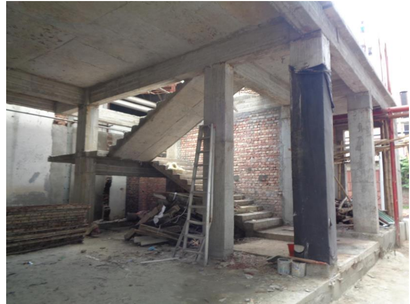
Lack of fall protection in the roof and open stair
