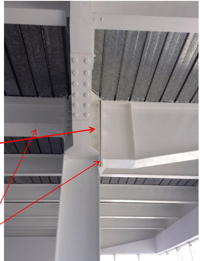
Connections between cantilevers on floor plate at level 2 appear light
