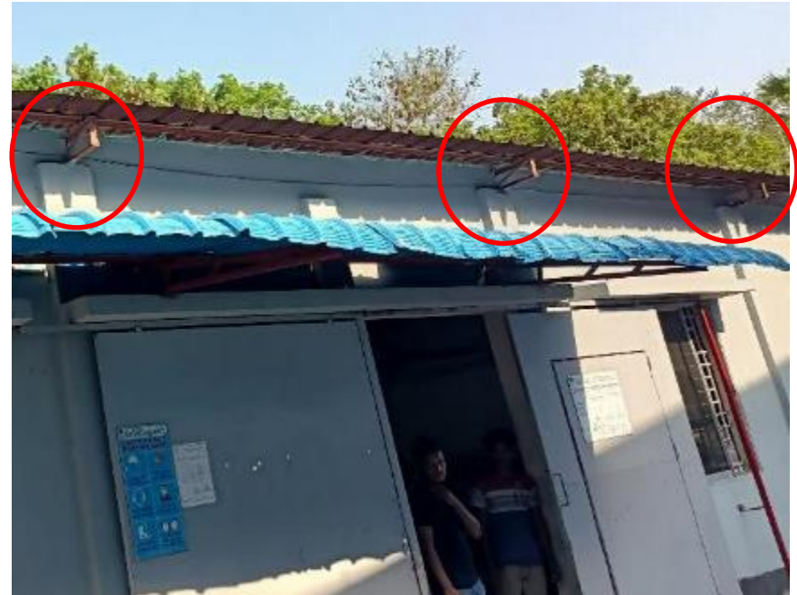
Truss connection with RC column
