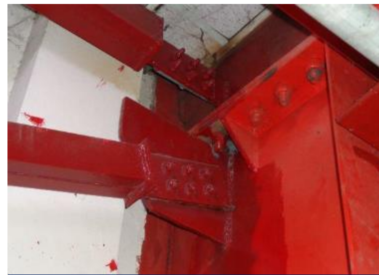
Strut and bracing
