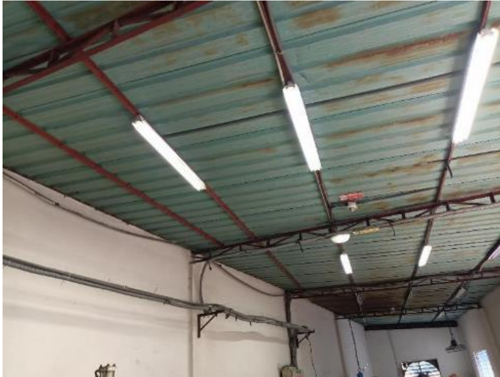
Inside of Poly Recycle Room
