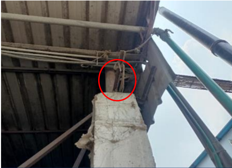
Truss connection with Steel column
