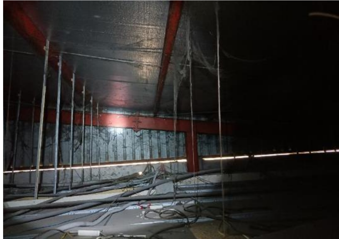
Rafter of grid 13
