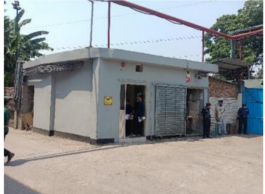
Security and Fire Pannel Room 2
