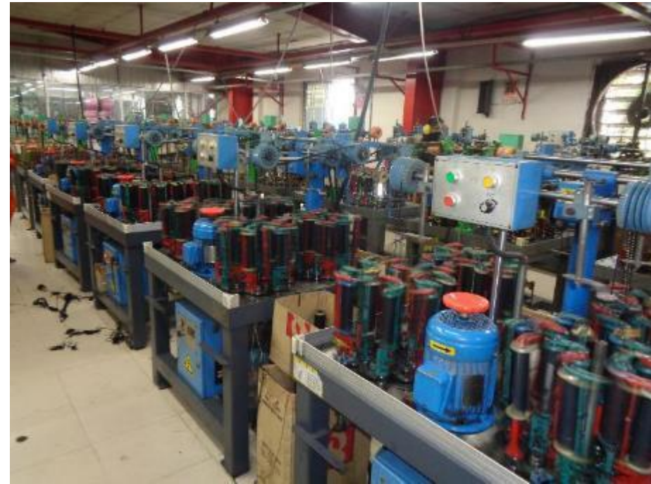
Vibration observed at the first floor
