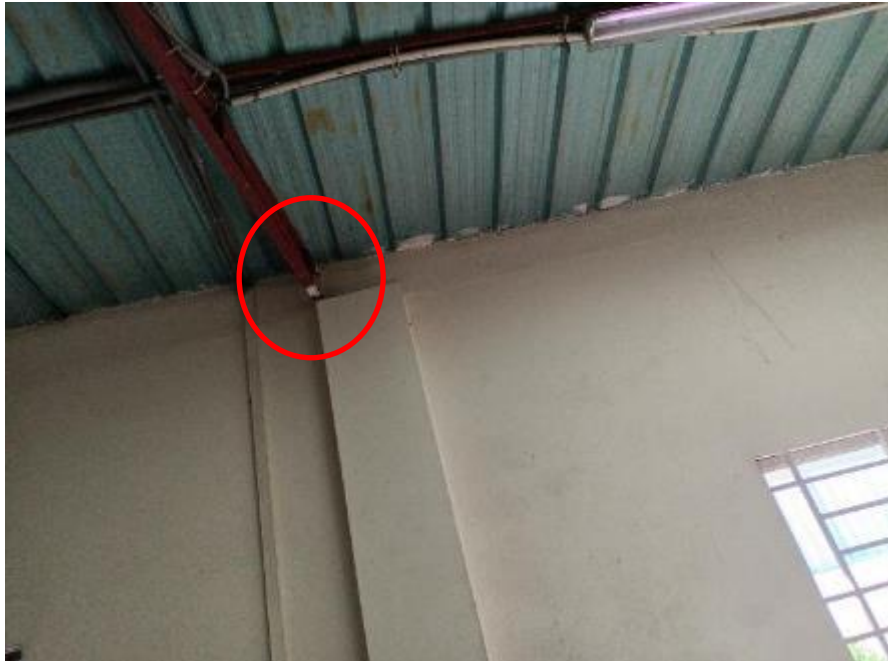
Truss connection with RC column
