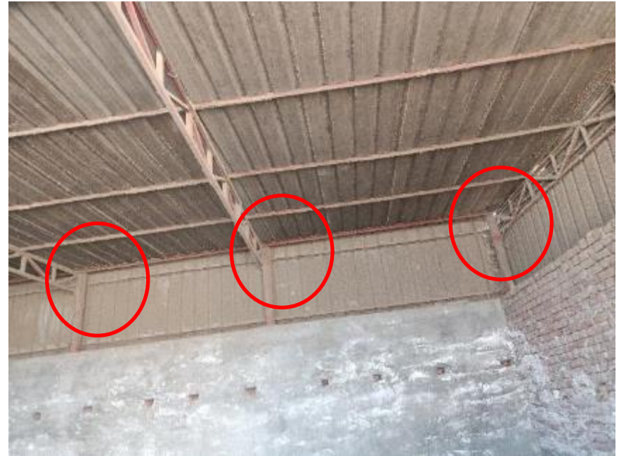
Truss connection with steel column
