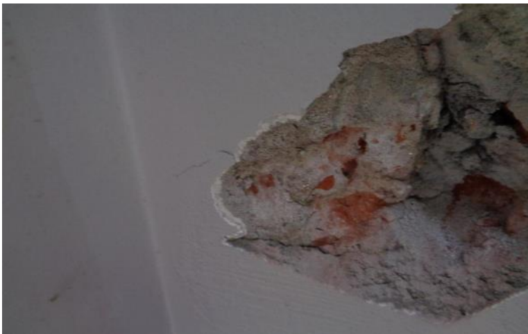
Dormitory Office Building : Brick aggregate
