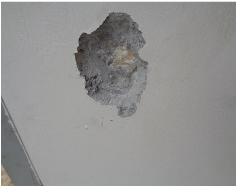
Utility Building : stone aggregate
