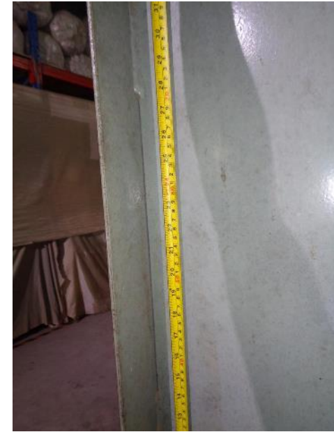
Tack welding- 350 mm spacing
