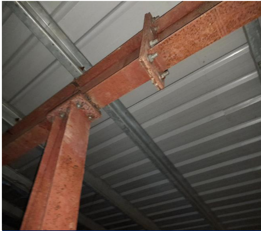
corroded steel member
