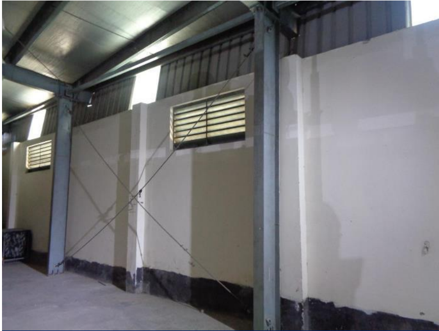
Loose cable bracing at wall and roof
