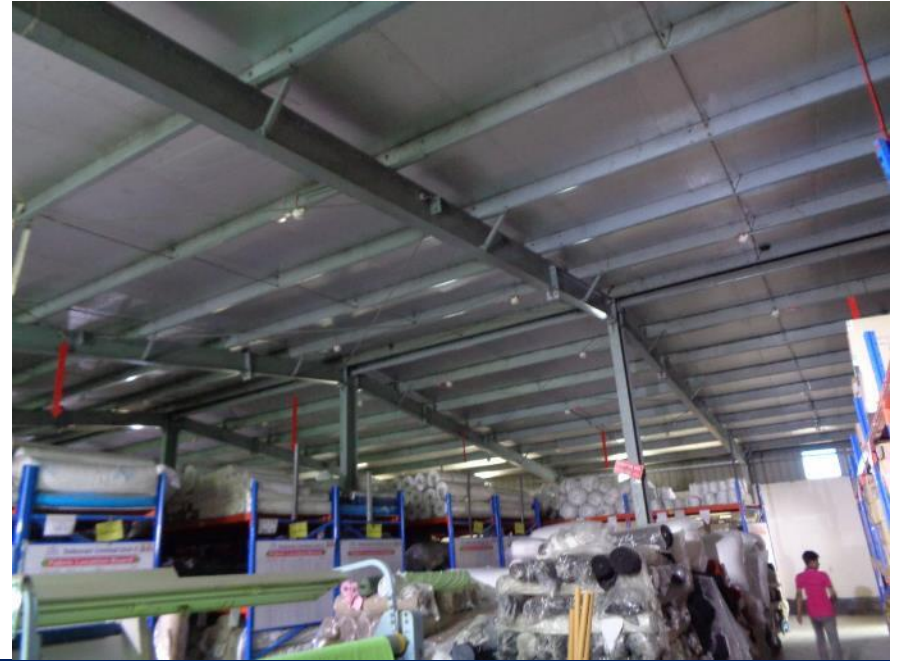
Loose cable bracing at wall and roof
