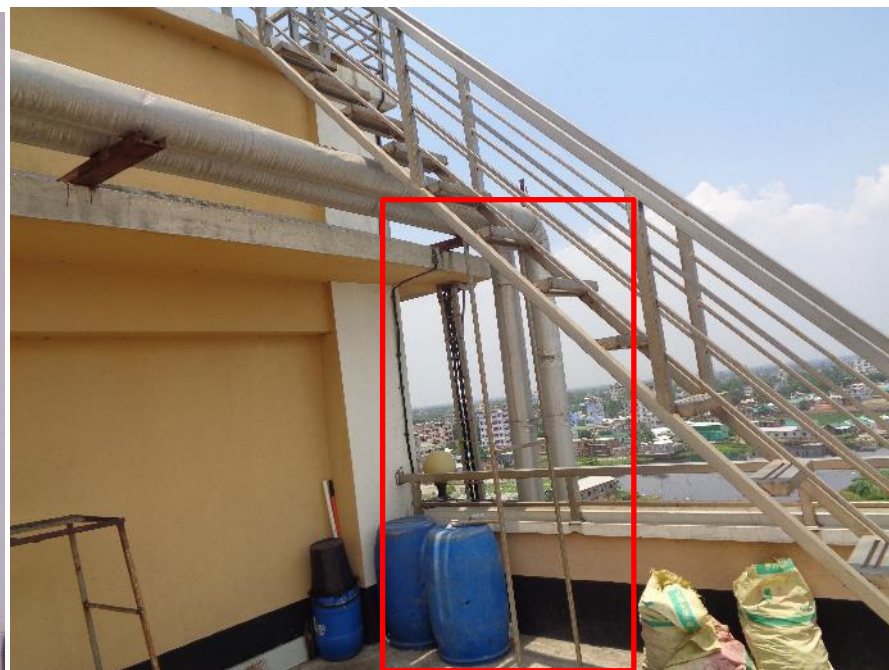
Support of ladder found as 20mmX20mm box
