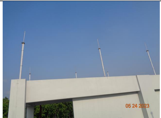
As-Built Lightning Protection System (LPS)
