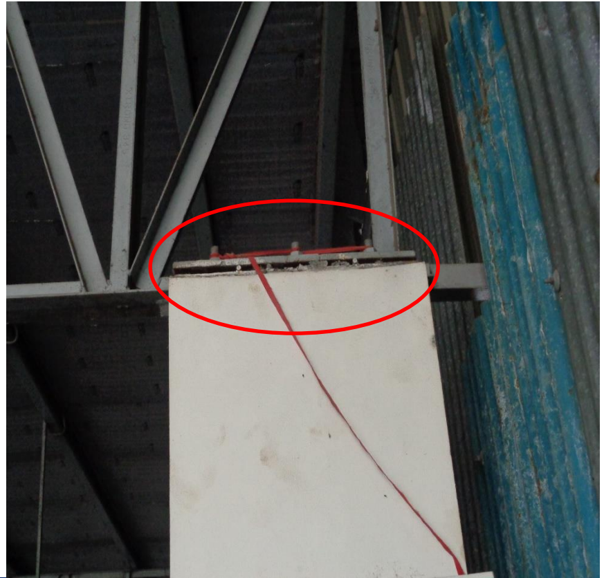
Gap between truss and RC column
