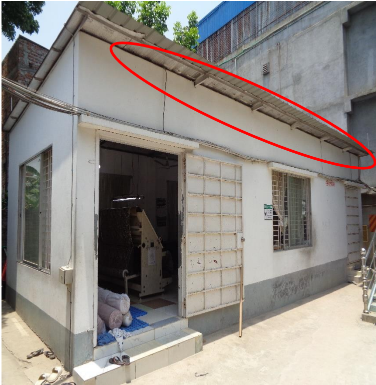
Steel rafters are inserted into brick wall
