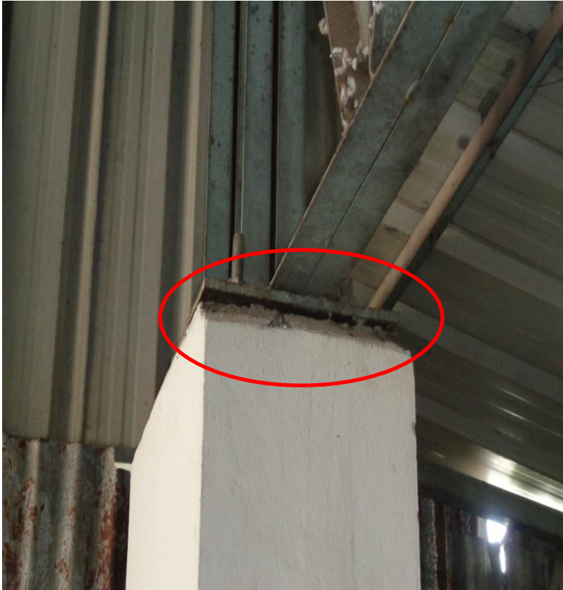
Gap between truss and RC column
