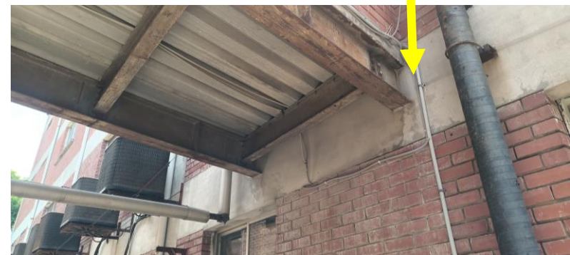
Connection with production building
