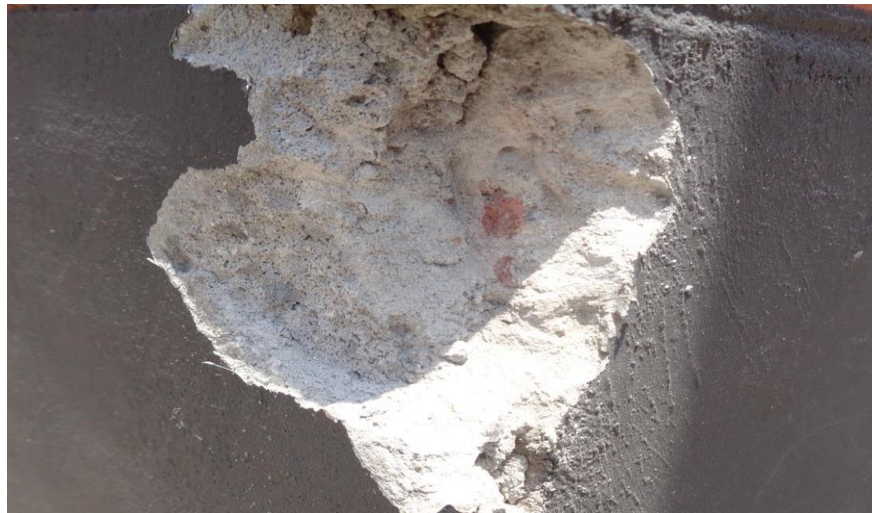
Substation Building: Brick aggregate
