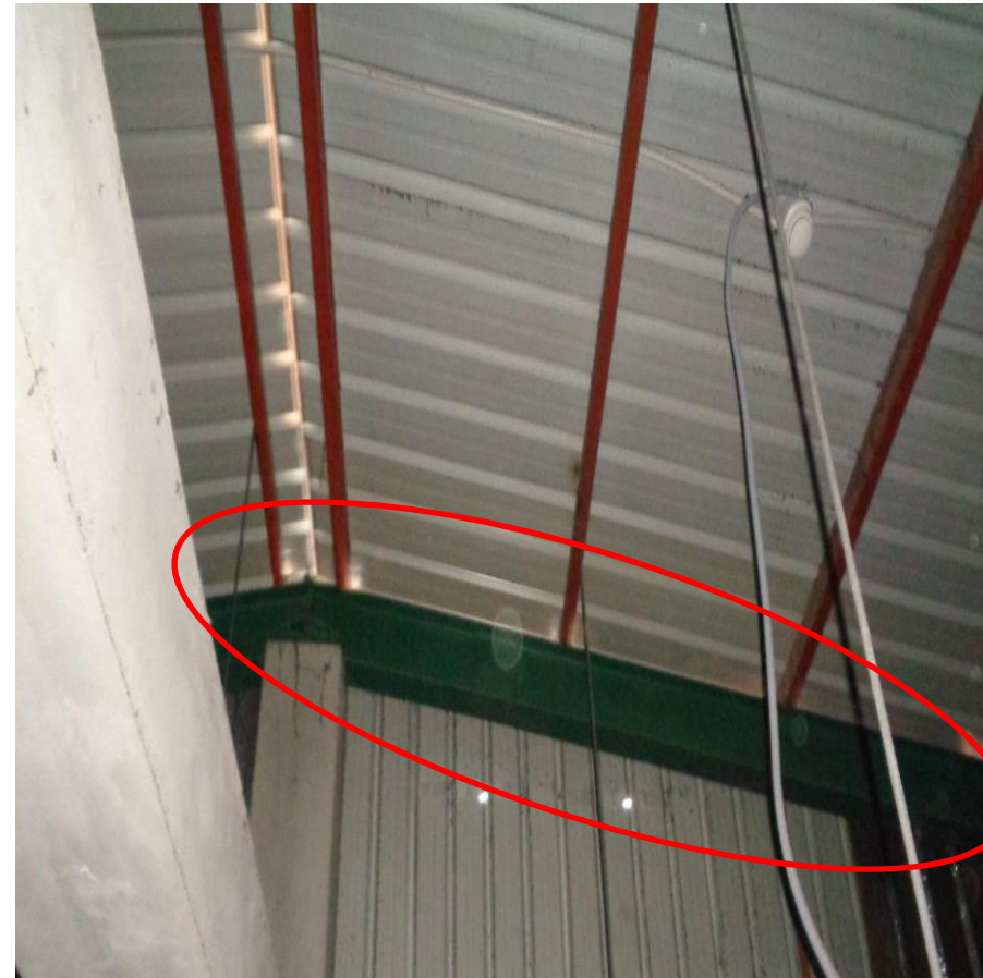
I-section rafter found onsite
