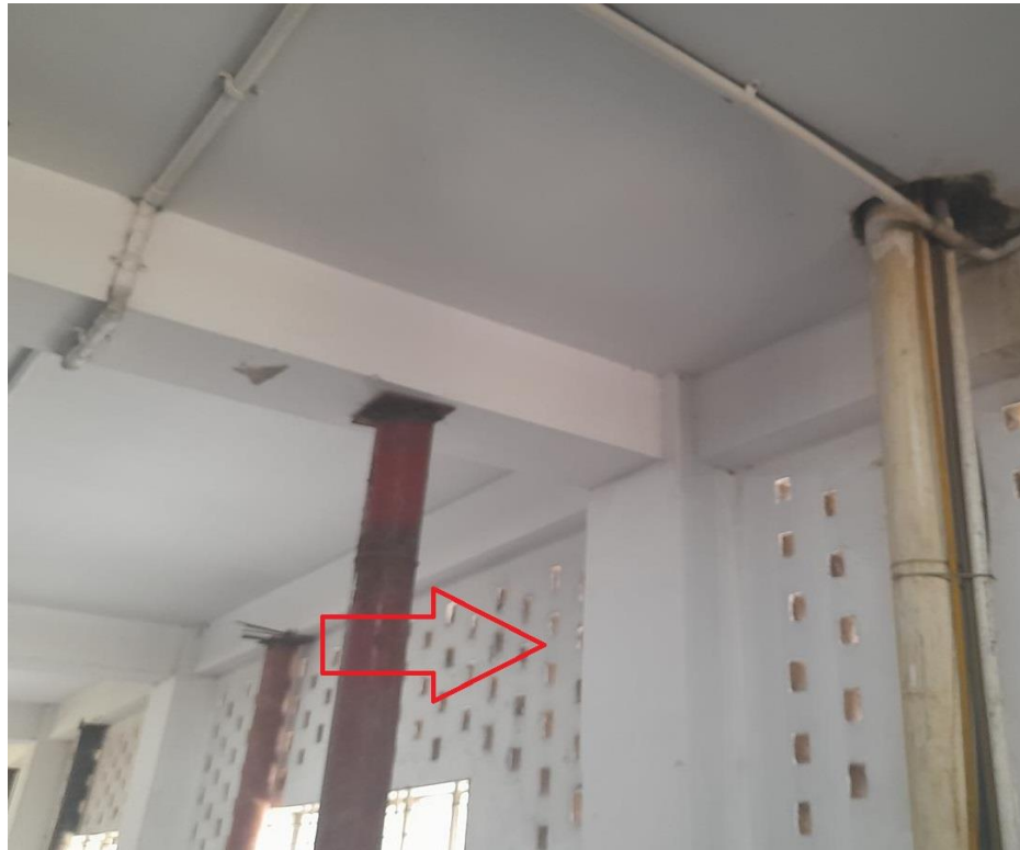
Locally repaired crack on column
