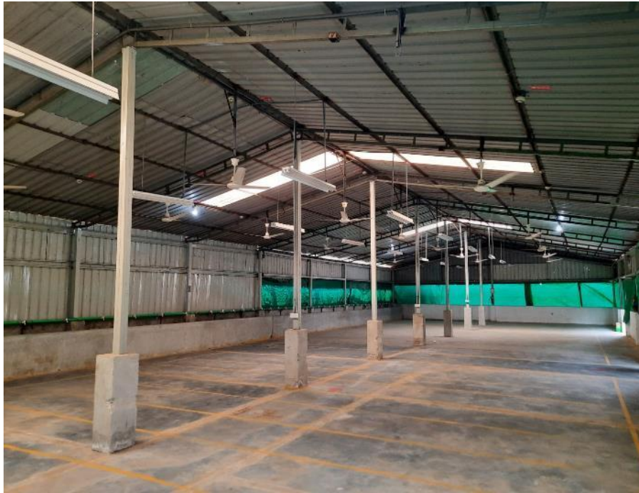
Only frame action in short direction
