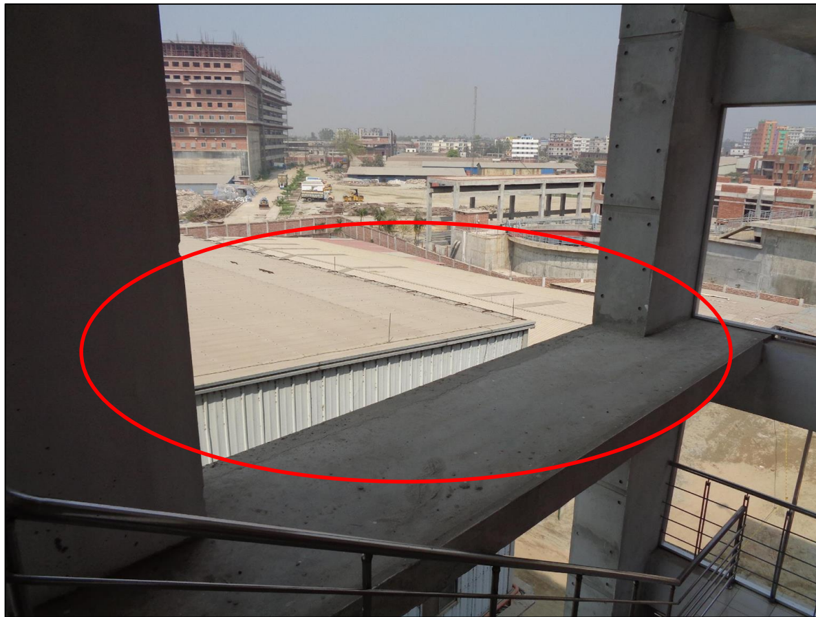
Opening at staircase
