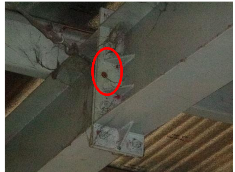
Bolt missing at several locations
