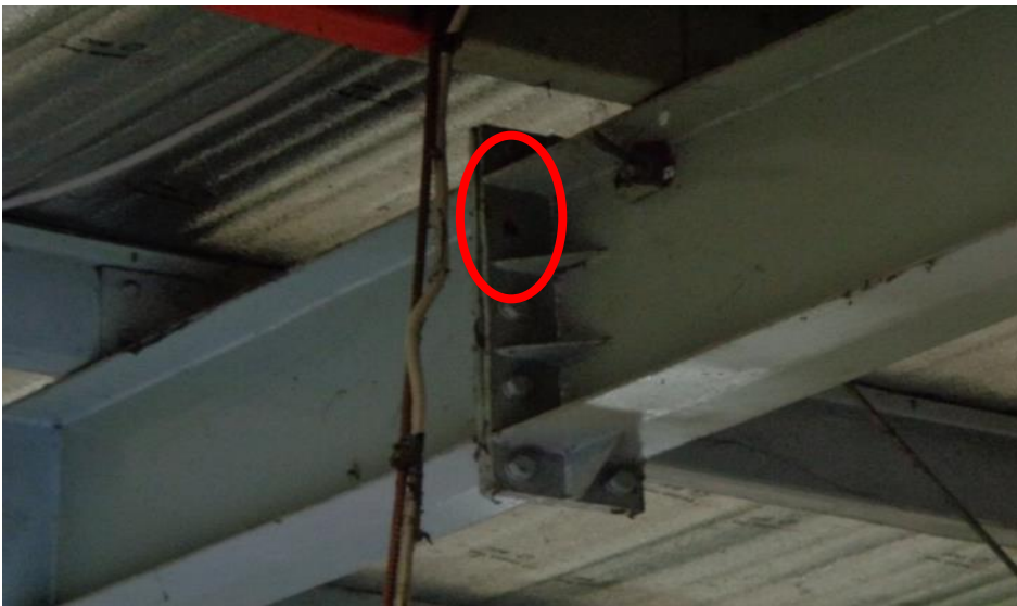
Bolt missing at several locations
