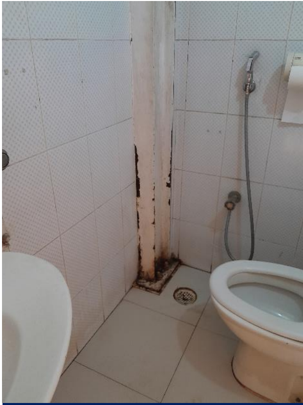
Corrosion (Inspection shed)
