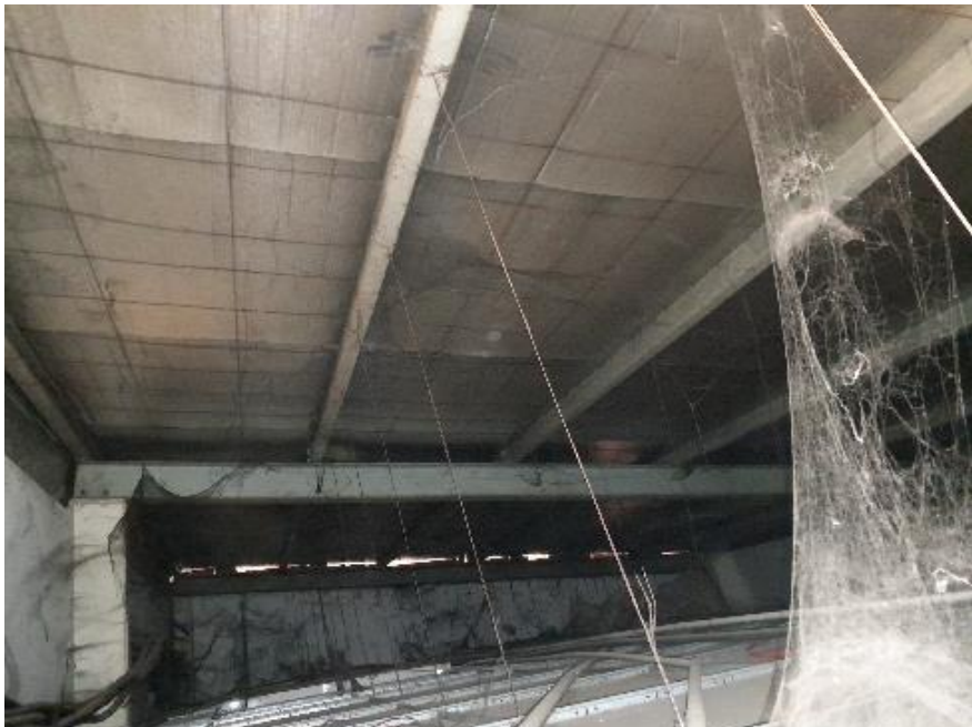
Absence of horizontal and vertical bracing at Inspection shed.
