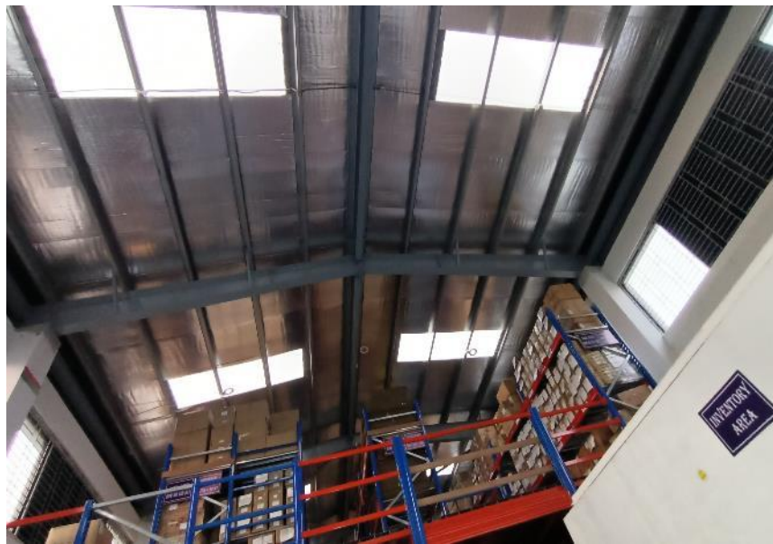
Inside of Store Shed
