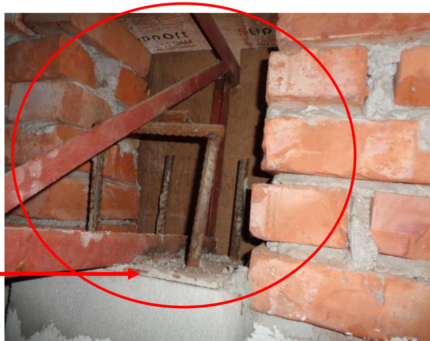
Connection with RC column
