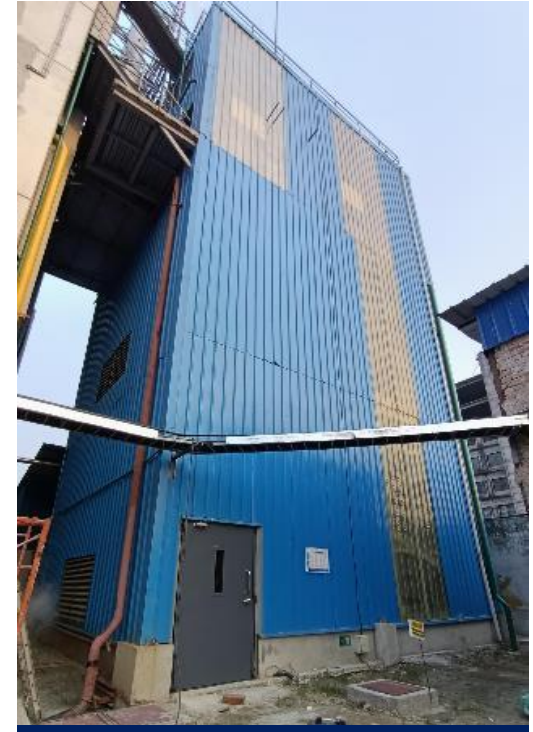
EGB Steel Building
