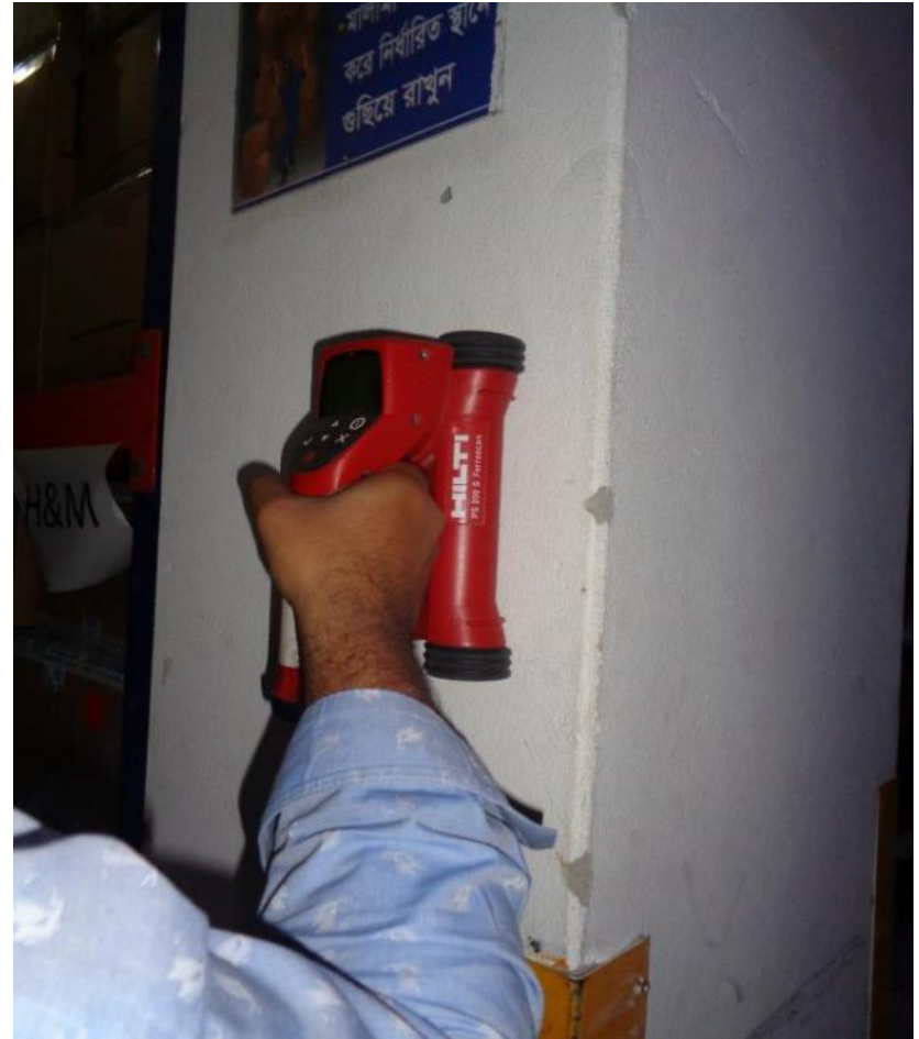
Rebar confirmed on-site by Ferro scan
