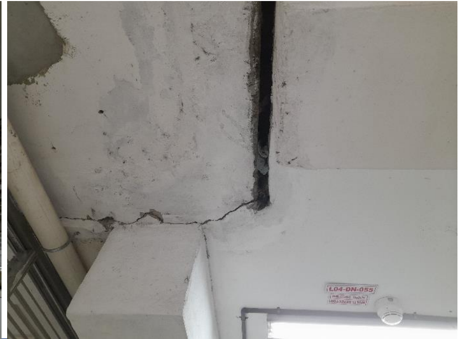
Loose material along the movement joints
