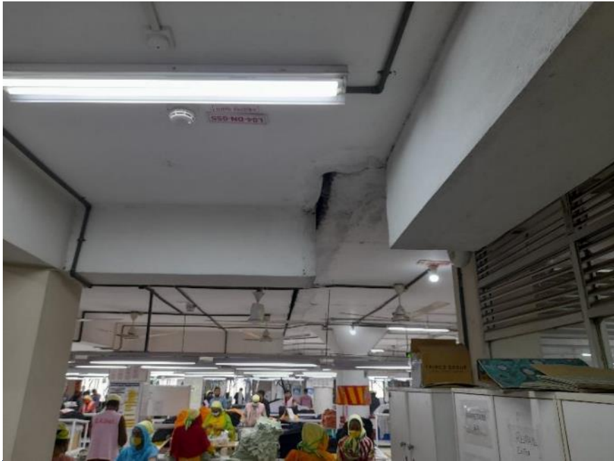
Loose material along the movement joints
