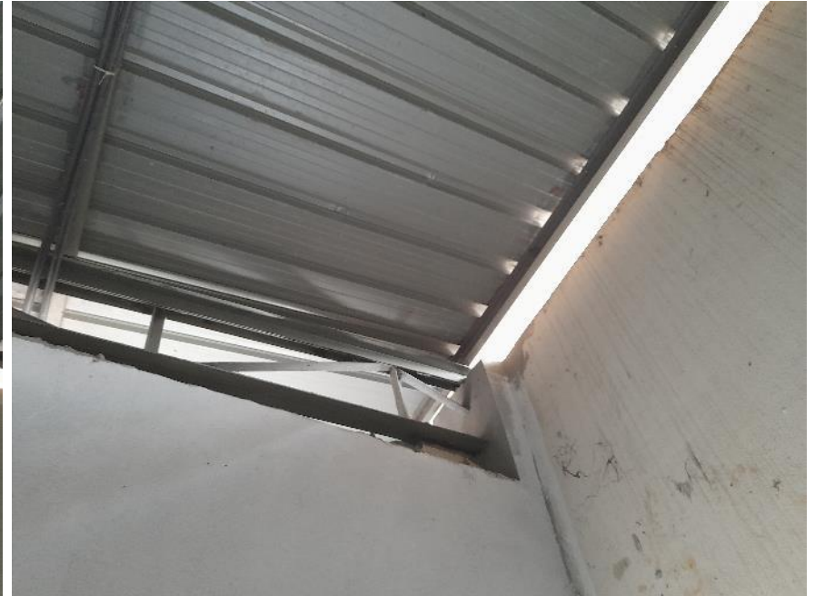
Truss to masonry wall connection
