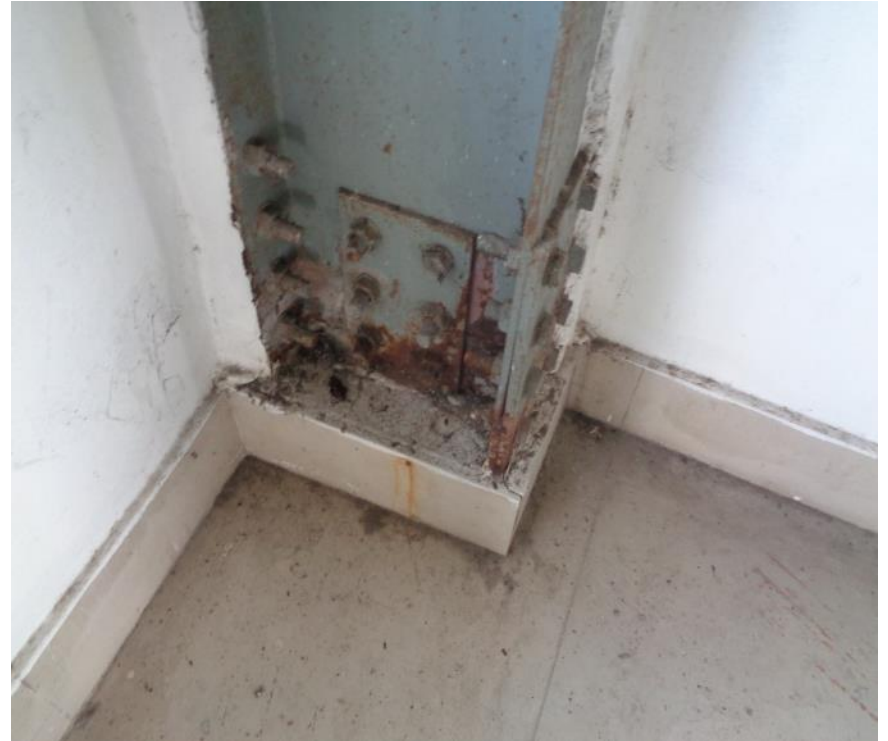
Severe corrosion in steel members
