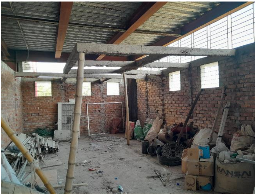
Unstable bamboo support on the demolition works which may slip away anytime.
