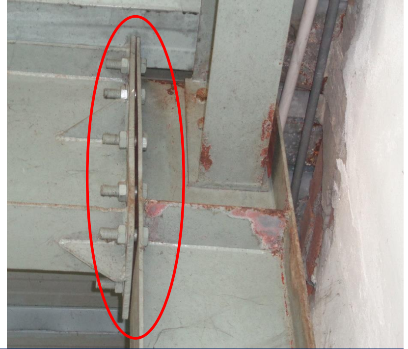
Significant gap in beam-column joint.
