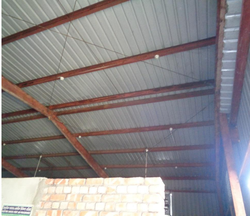
Roof bracing is provided at some locations
