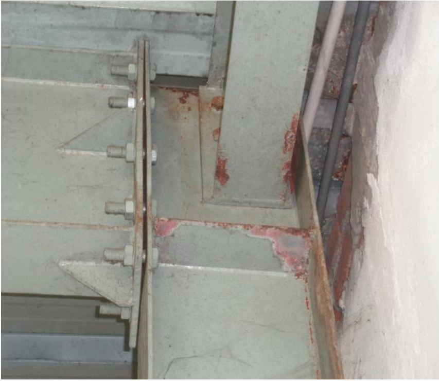
Severe corrosion in steel members
