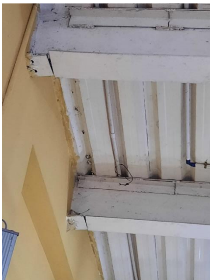
Faulty retrofitting works (disconnected flange).
