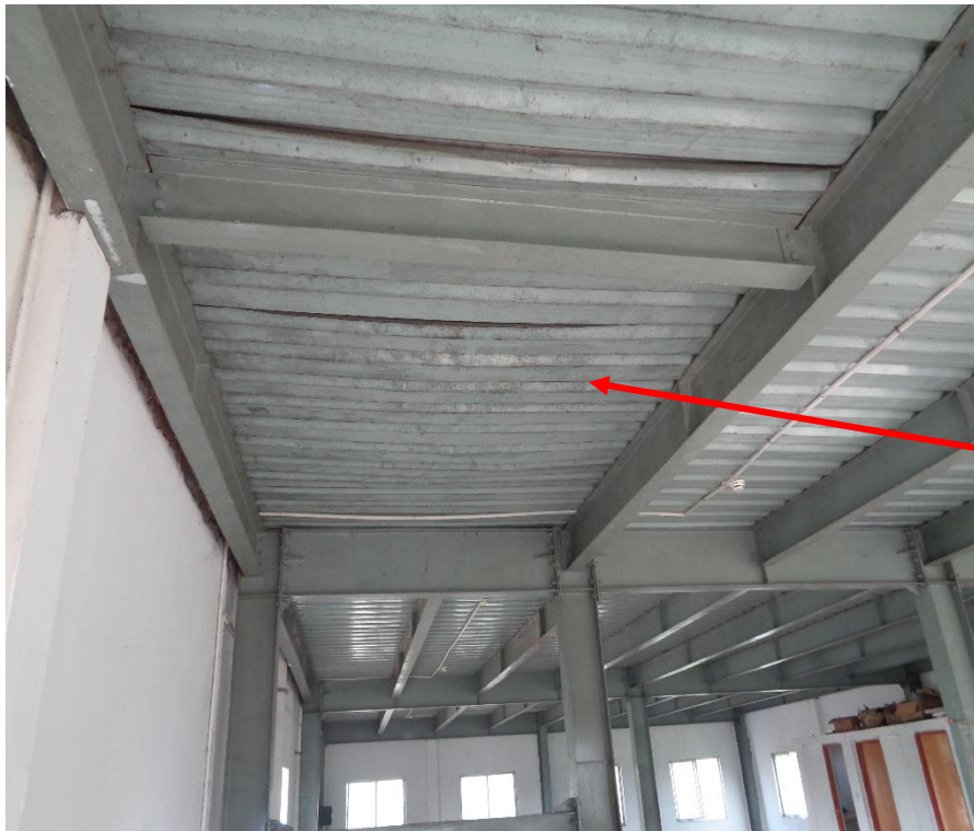
Deflection in steel deck slab (roof)
