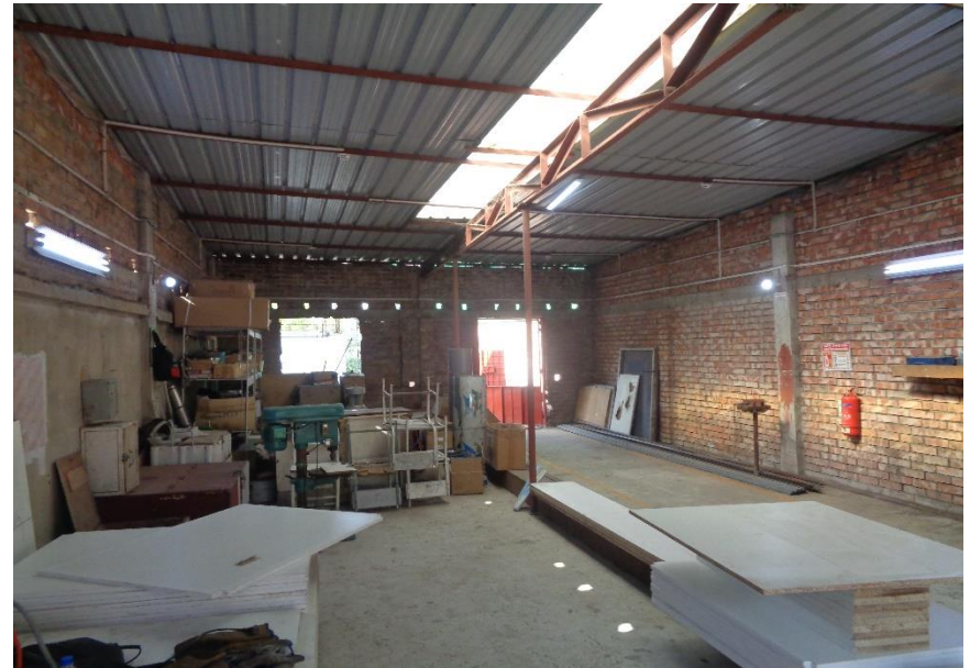
Purlin inserted to brick wall
