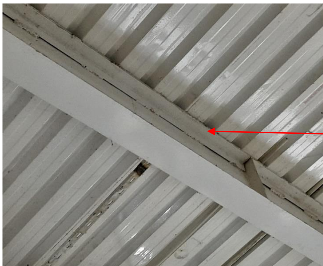
Tack welding found instead of continuous welding at steel column and beam retrofitting
