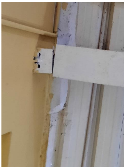
Faulty retrofitting works (disconnected flange).
