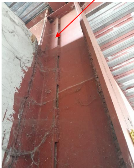
Tack welding found instead of continuous welding at steel column and beam retrofitting
