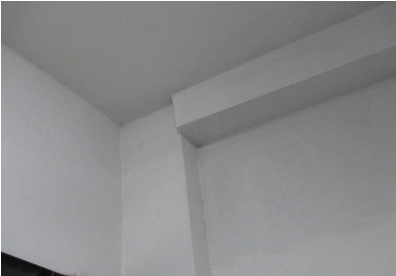
Beam and column joint on 2 nd floor
