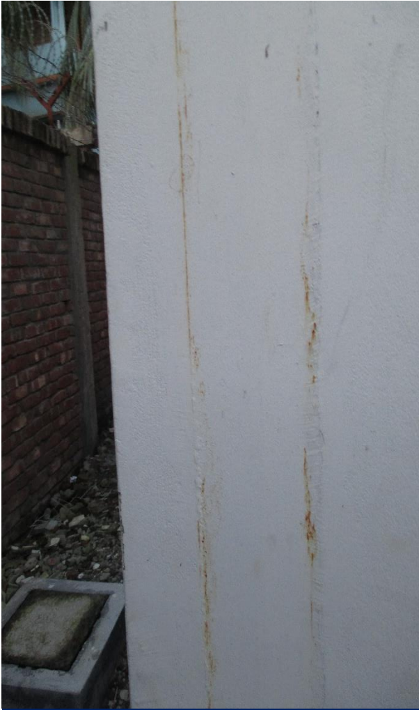
Steel corner Column
