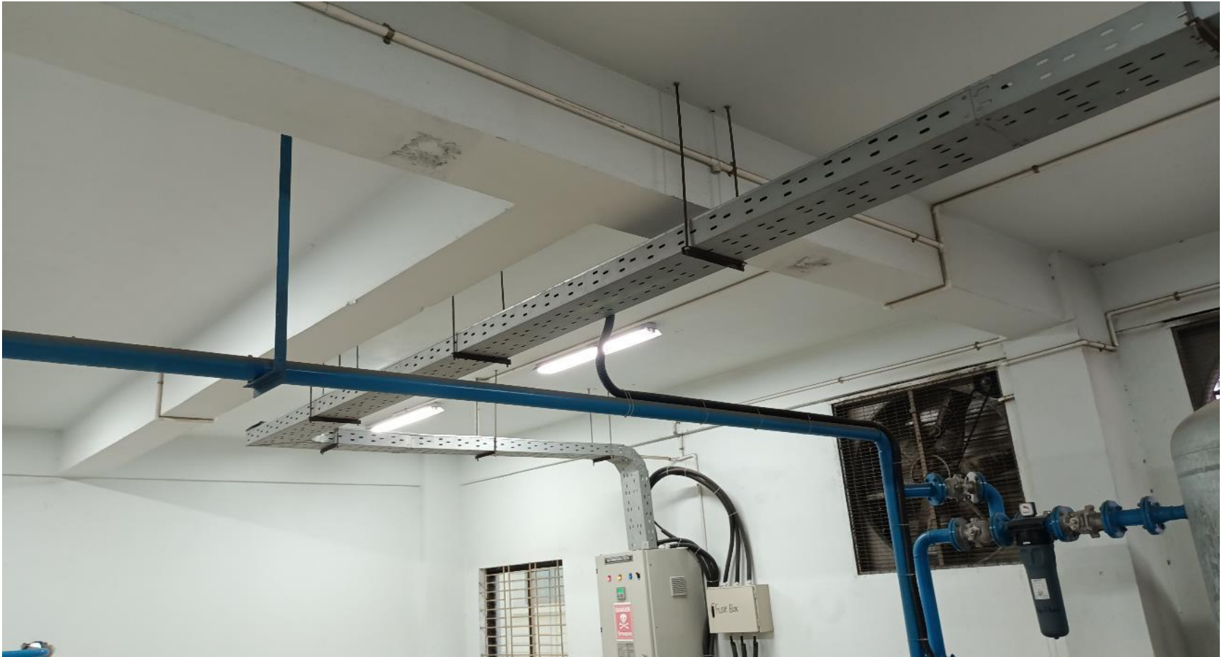
First floor beam
