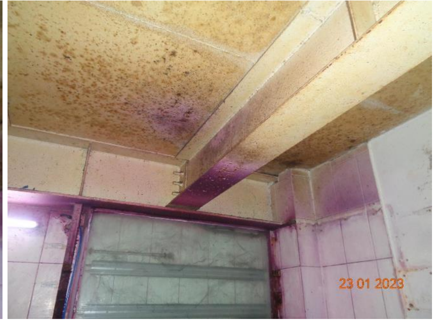
Appearance of corrosion in steel members
