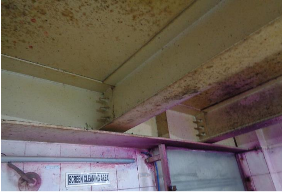
Appearance of corrosion in steel members
