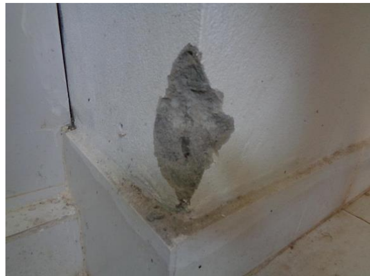
Stone aggregate in retrofitting column of Building-5
