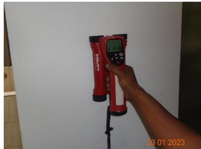
Rebar checked by ferro scanner
