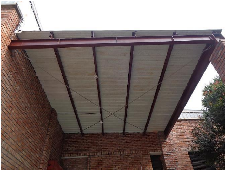
The rafter of loading-unloading zone
