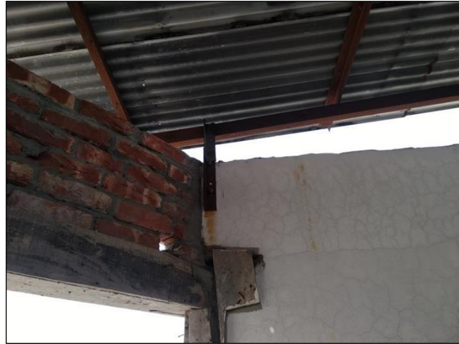
Corrosion in the steel members of the RO plant at rooftop.
