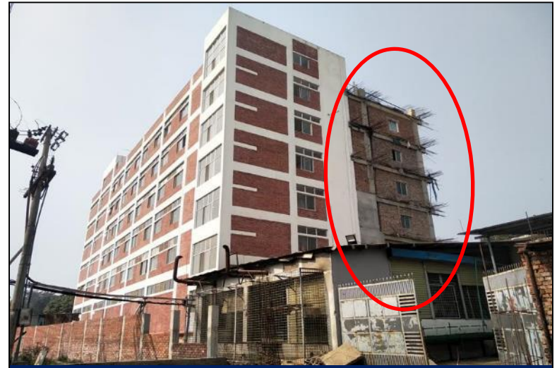
Exposed rebar kept at east side for horizontal extension
