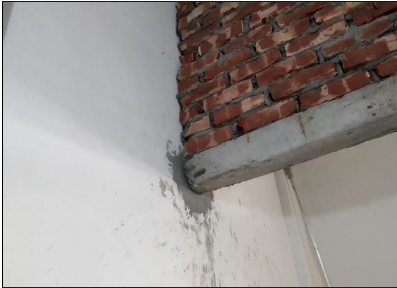
Inadequate lintel support at toilet zone
