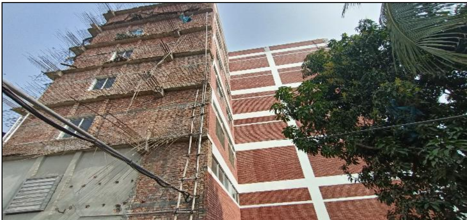
Exposed rebar kept at west side for horizontal extension
