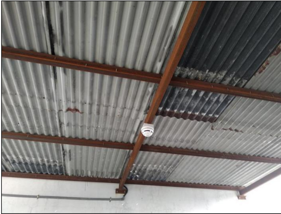
Corrosion in the steel members of the RO plant at rooftop.
