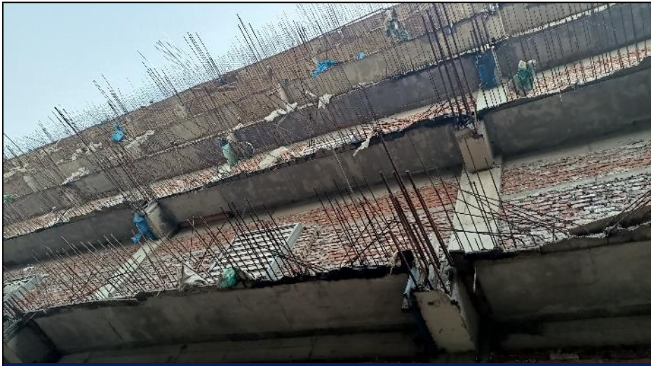
Exposed rebar kept at north side for horizontal extension
