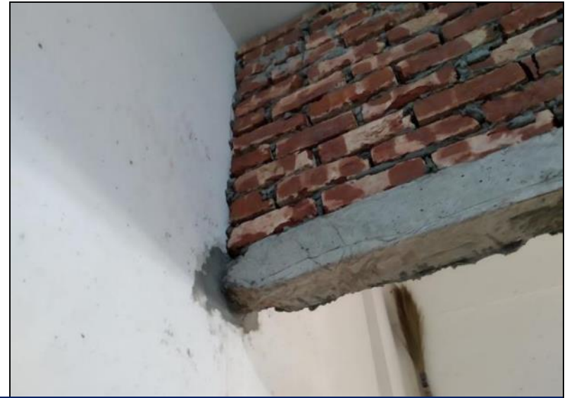
Inadequate lintel support at toilet zone
