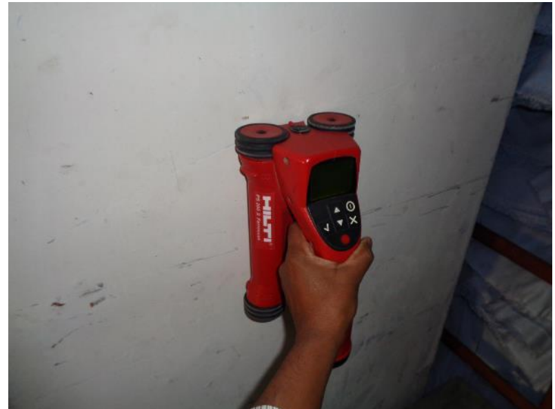
Rebar checked by ferro scanner
